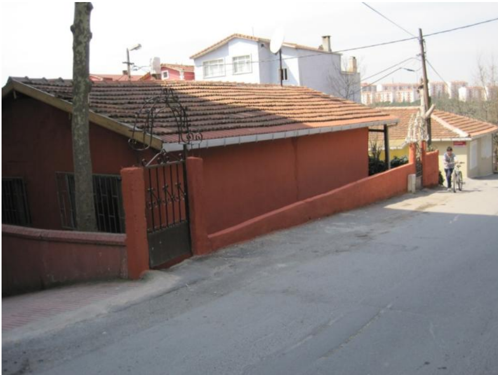
Figure 7.18: Low-rise buildings near edge of neighborhood – Fatih Sultan Mehmet
