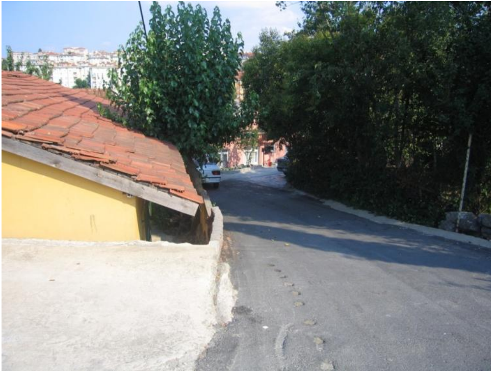
Figure 6.11: Buildings and roads adapting to topography Karanfilköy
