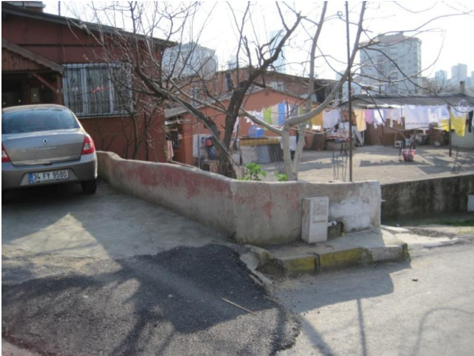
Figure 7.13: Low-rise buildings near edge of neighborhood - Karanfilköy
