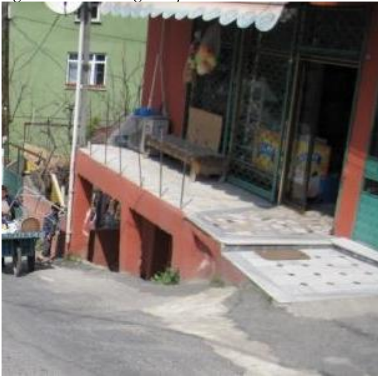
Figure 6.23: Building adapted to the terrain - Fatih Sultan Mehmet
