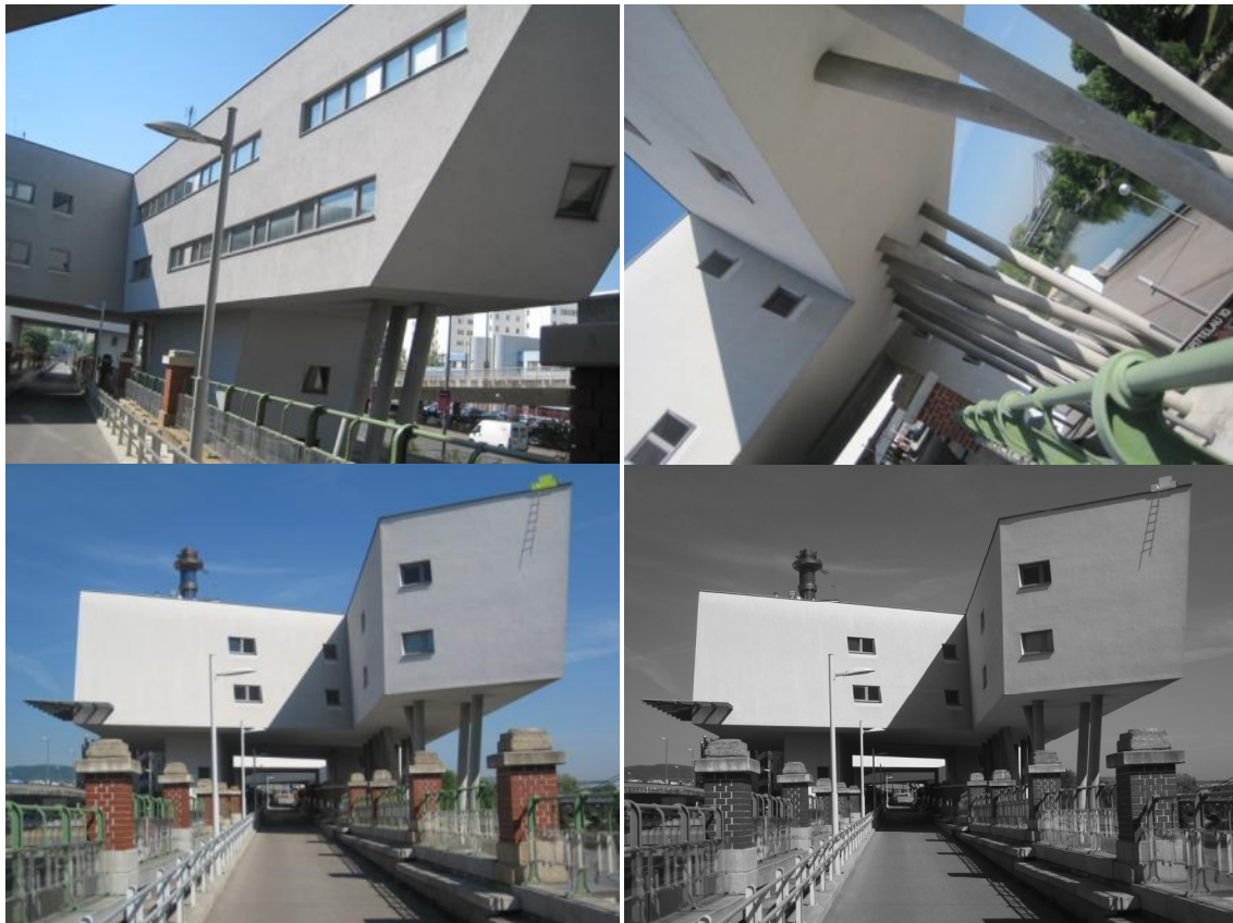
Figure C.3: Spittelau Viaducts Housing Project – Vienna, Austria
