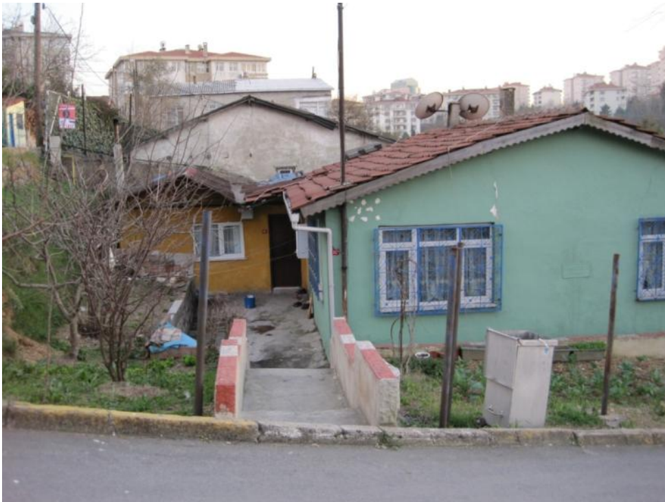
Figure 7.15: Low-rise buildings near edge of neighborhood - Karanfilköy
