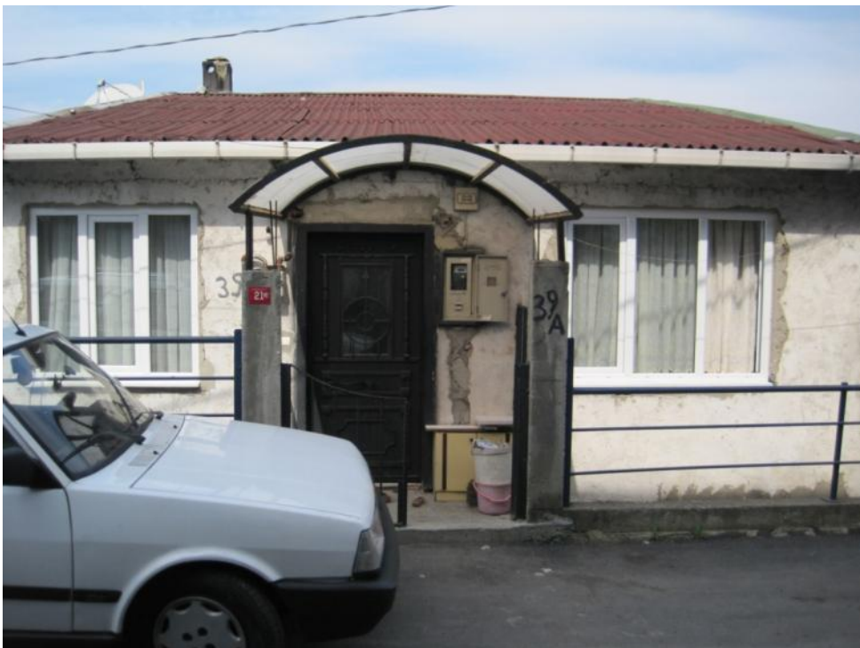
Figure 7.16: Low-rise buildings near edge of neighborhood – Fatih Sultan Mehmet
