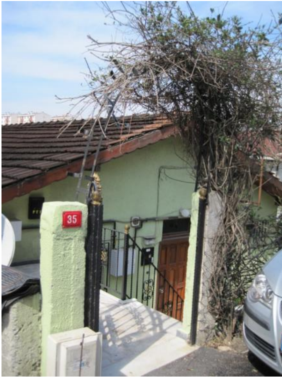
Figure 7.17: Low-rise buildings near edge of neighborhood – Fatih Sultan Mehmet
