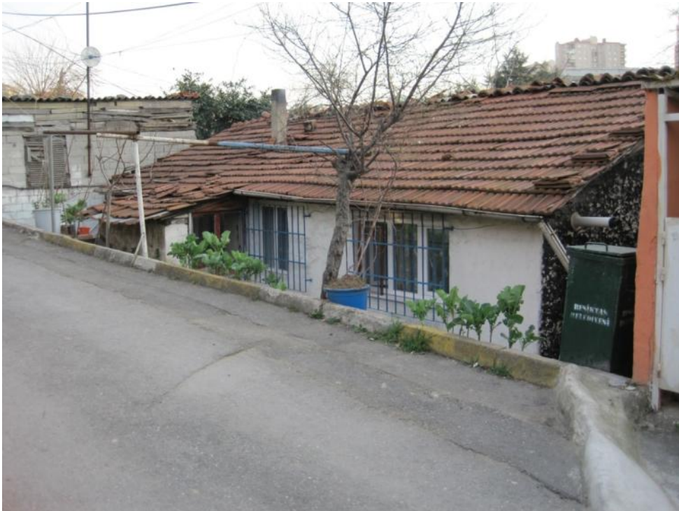
Figure 7.14: Low-rise buildings near edge of neighborhood - Karanfilköy
