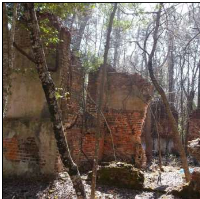
Figure 114. Riverside elevation, eastern extent, showing missing sections of wall.
