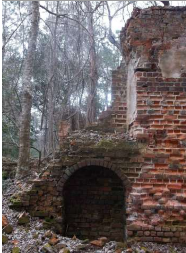
Figure 43. West elevation, interior wall with relieving arch.
