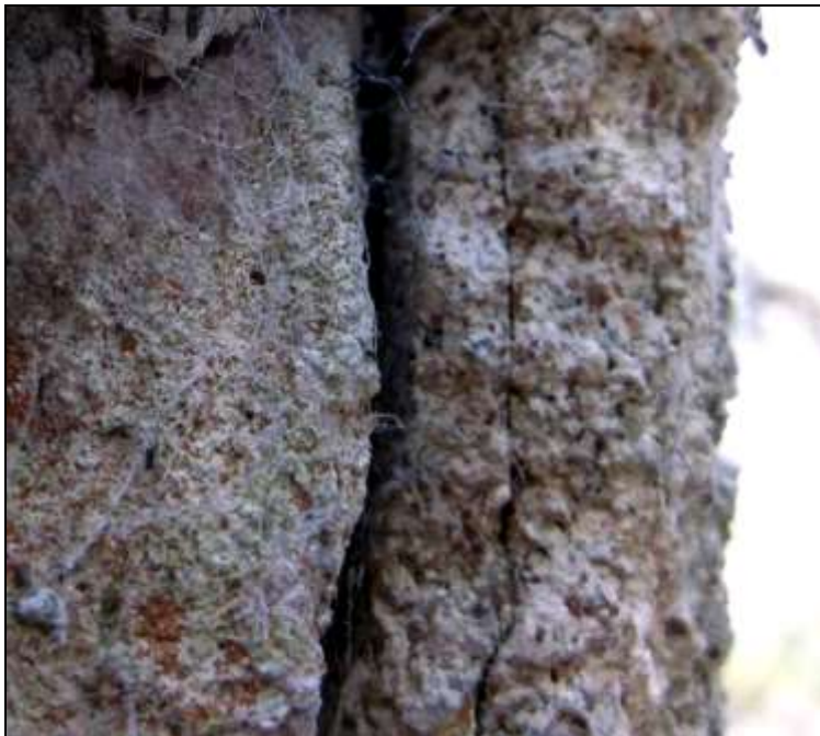
Figure 22. Close-up photo of stucco in three coats.
