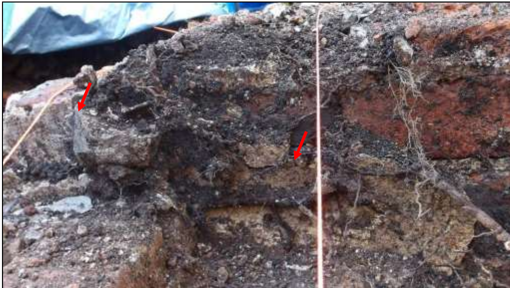
Figure 68. Close-up of remnant plaster on the north-south wall behind the chimney flue.
