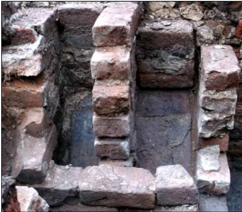
Figure 73. Close-up of chimney flues.
