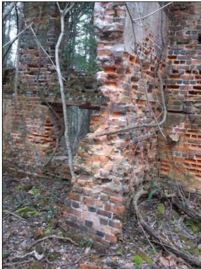
Figure 46. East elevation, interior T-wall.
