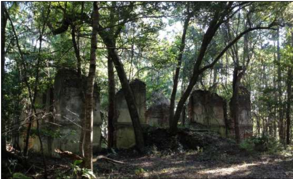
Figure 1. Peachtree Plantation, landside elevation; view southeast.
