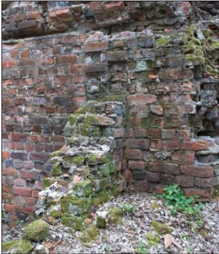
Figure 48. Interior riverside elevation, west side showing interior wall remnant.
