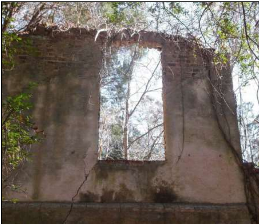
Figure 36. Segmental arch at the northern extent of the west elevation.
