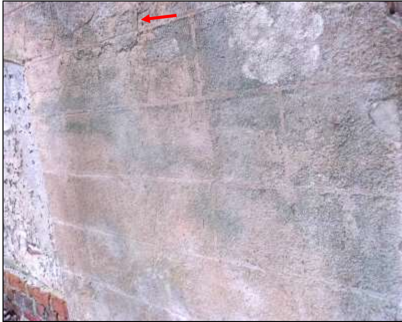
Figure 20. Riverside elevation showing a section of stucco with possible repair.
