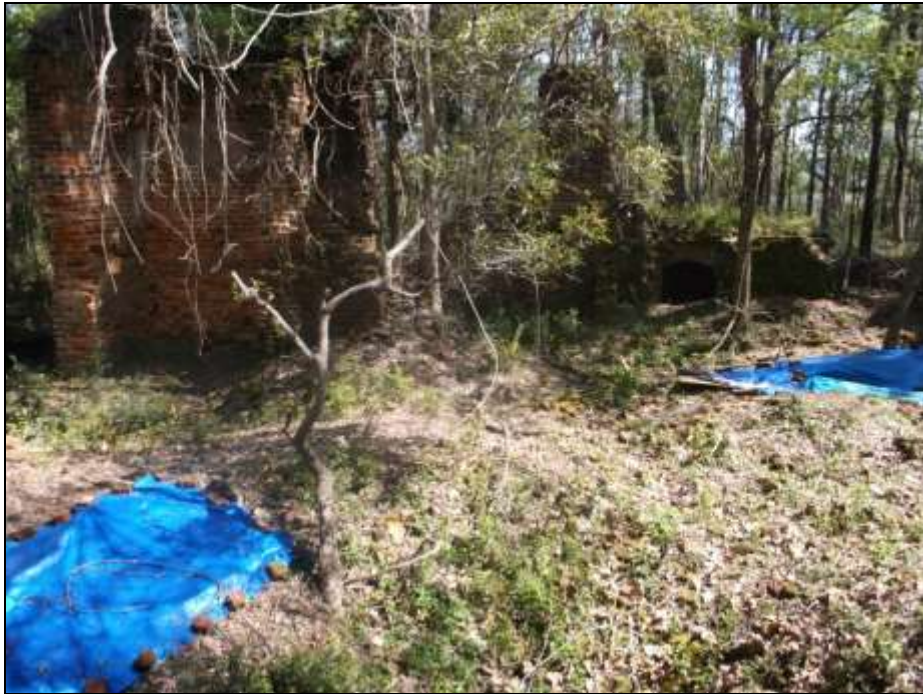
Figure 38. Interior of Peachtree showing wall remnants on the west elevation.
