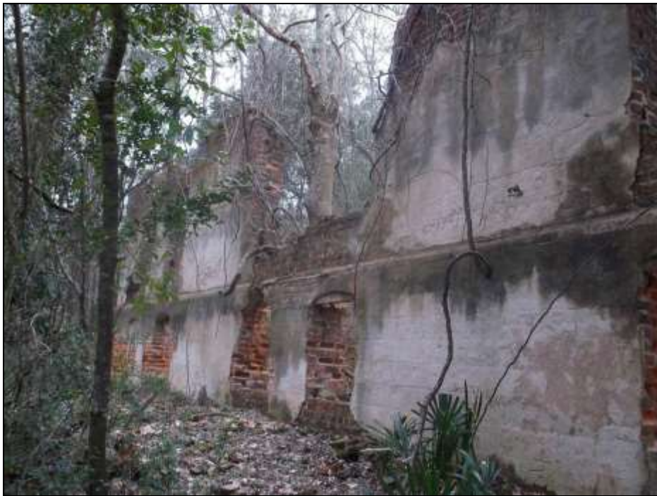
Figure 106. Overview of east elevation, central bays; view west.
