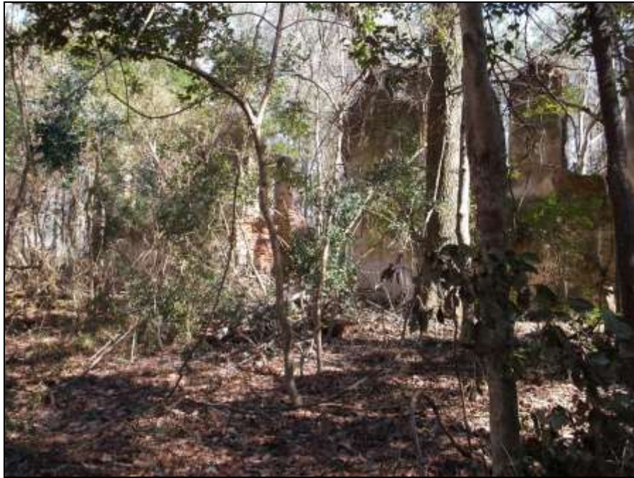
Figure 35. West elevation overview.
