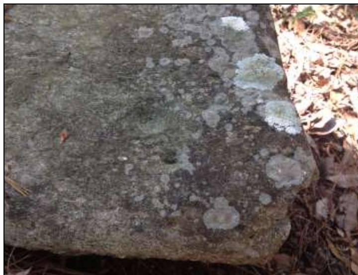
Figure 33. Close-up of riverside portico stair showing the ghost mark of a balustrade.
