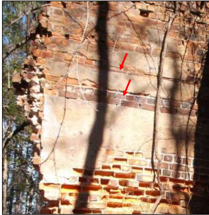
Figure 52. Ghost marks of shelving, interior wall, east elevation.
