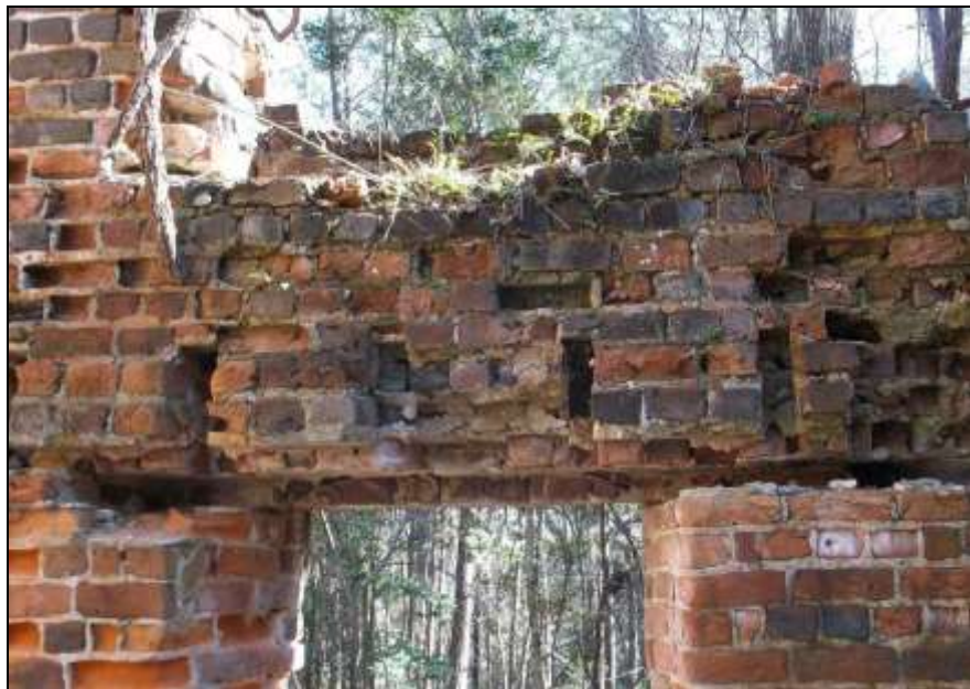
Figure 49. East elevation interior, northern extent showing joist and window sill pockets.
