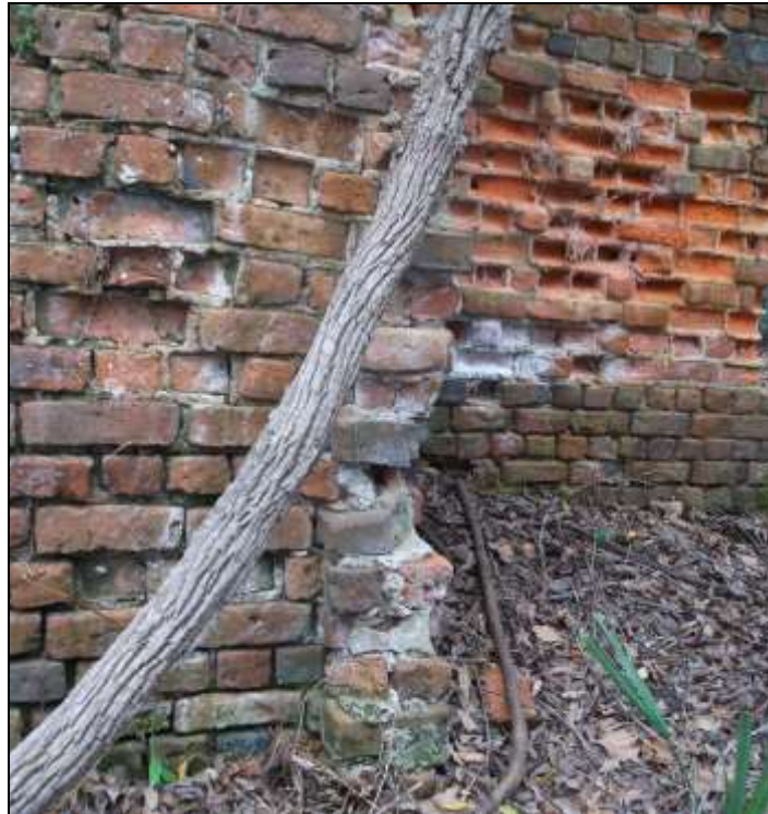
Figure 47. Interior landside elevation, west side, showing the remnants of a smaller wall.
