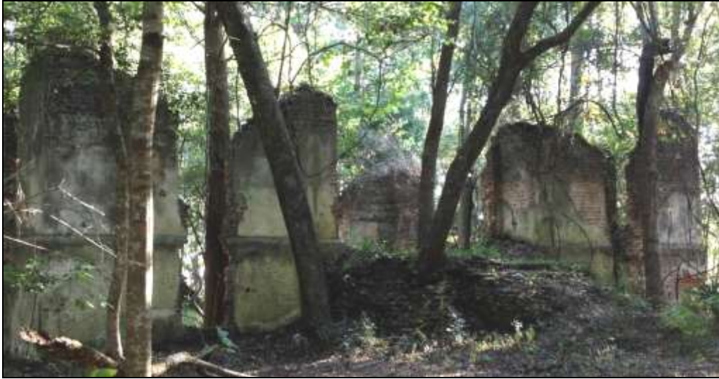
Figure 26. The landside elevation and portico, 2013.
