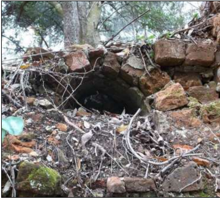
Figure 41. Close-up of drainage remnant, interior landside elevation, western extent.
