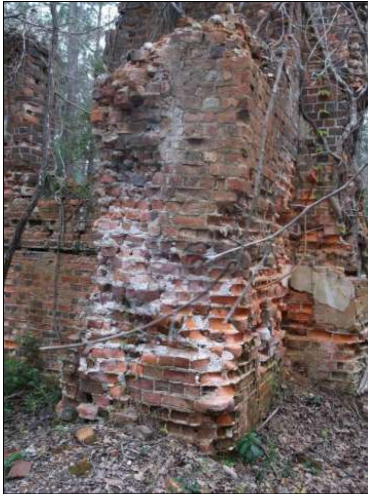
Figure 42. West elevation, interior remnant flue stack.
