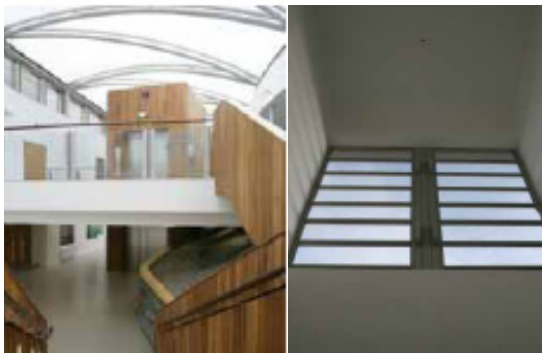
Figure 83: Main atria with glass roof and clerestories along corridor of inpatient unit.
