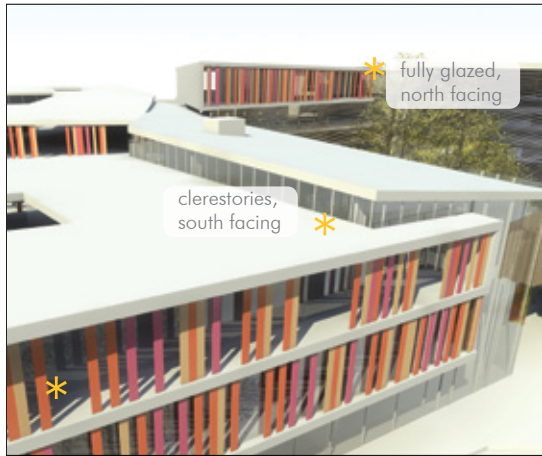
Figure 150: Clerestories on southern side of circulation spine provide direct sunlight for the space.
