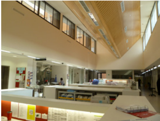
Figure 117: High clerestories in Intensive Care Unit for effective daylight penetration, Alfred Hospital, Melbourne, Australia.
