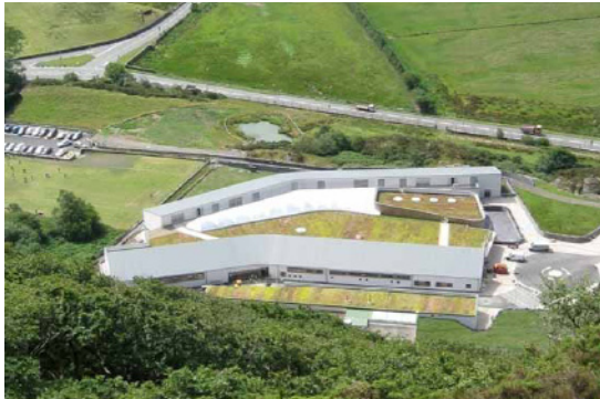
Figure 82: Narrow building footprint of Alltwen Community Hospital.
