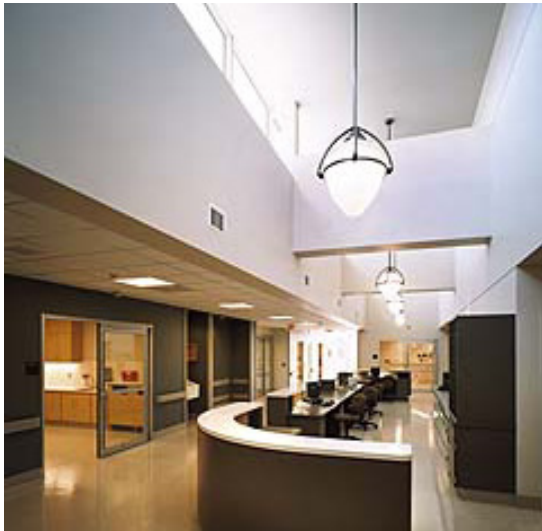
Figure 114: Clerestories above nurse station of ED, St. Mary's Hospital, Walla Walla, US
