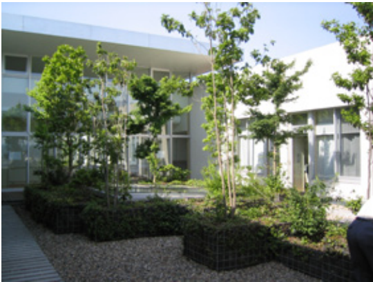
Figure 110: Skylights at the bottom of courtyards provide daylight for the story below.
