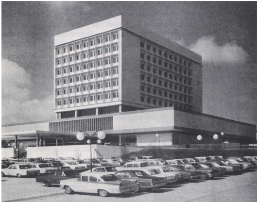
14. The modern aesthetic characteristic of hospitals from the Hill-Burton era.
