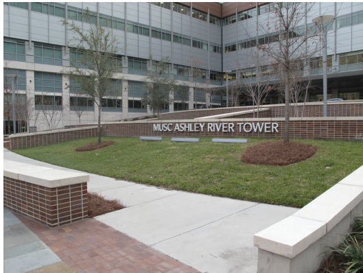
6. Front entrance of the new MUSC Ashley River Tower.
