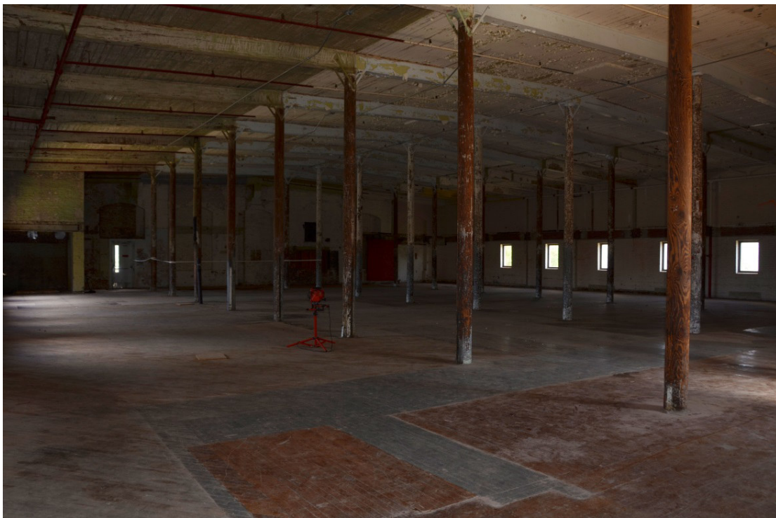
Figure 3-11. Image showing the Sorting Room at the Cigar Factory, Charleston, South Carolina. Historic mills used vast expanses to house large quantities of goods and facilitate easy movement through the spaces. Photo by author.
