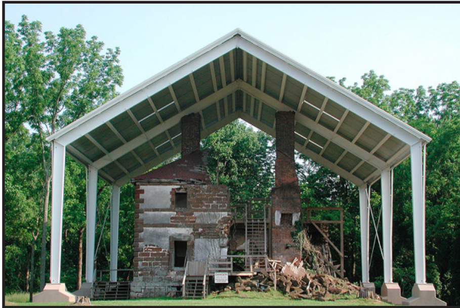
Figure 23. Image Showing the Shelter over Menokin circa 2000 (Menokin Foundation).
