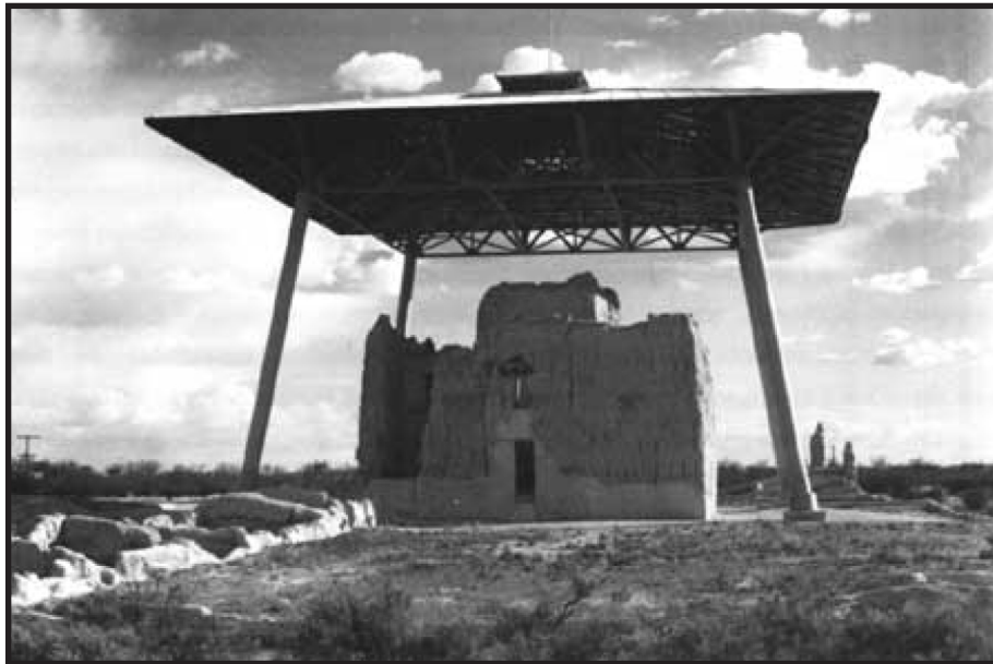
Figure 22. Image Showing the Current Shelter over Casa Grande circa 1932 (National Park Service, www.nps.gov ).
