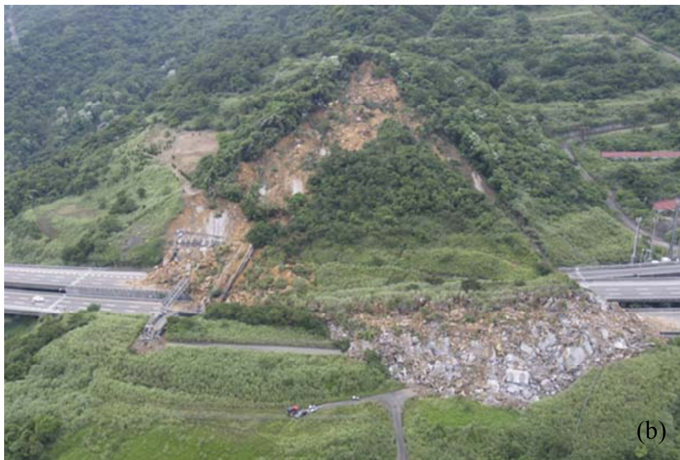
Figure 2.1: Site photograph of the Freeway No.3 landslide in Taiwan: (a) Panoramic view; (b) Another view (National Airborne Service Corps, Ministry of Interior, Taiwan, 2011, http://www.nasc.gov.tw/ )
