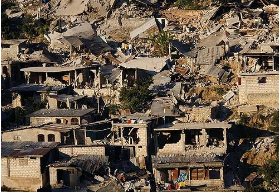
Figure 2.2 Earthquake damage (LA Times)
