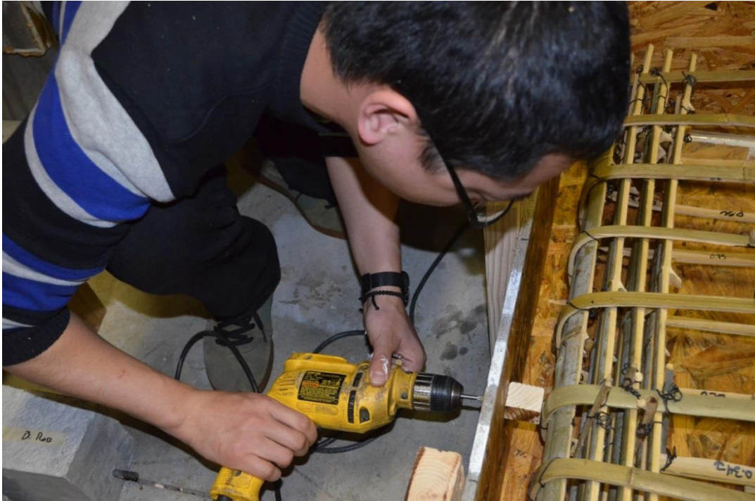
Figure 6.22 Installation of block spacers
