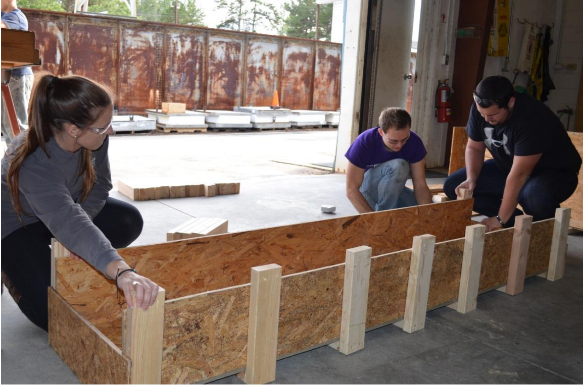
Figure 6.21 Beam formwork preparation
