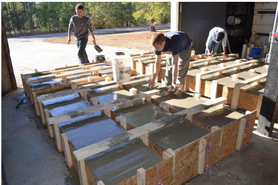
Figure 6.25 Finishing concrete with a steel finishing trowel
