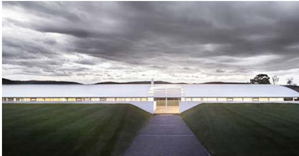
Figure 38: front elevation of Spencertown House, with retaining wall and view through (edit Braden Reid)
