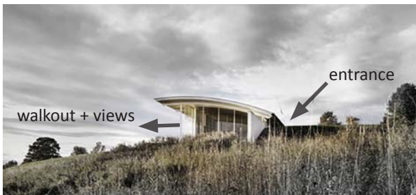
Figure 40: side elevation of Spencertown House showing placement in topography (edit Braden Reid)
