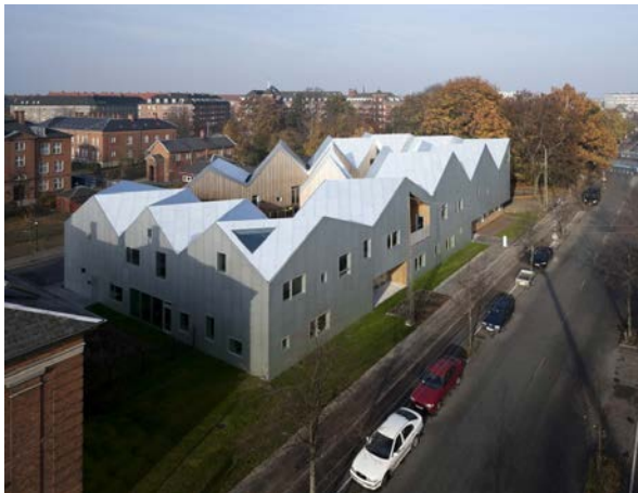
Figure 22: birdseye view of the Centre for Cancer and Health in Copenhagen, in contrast to its red brick surroundings (NORD Architects)
