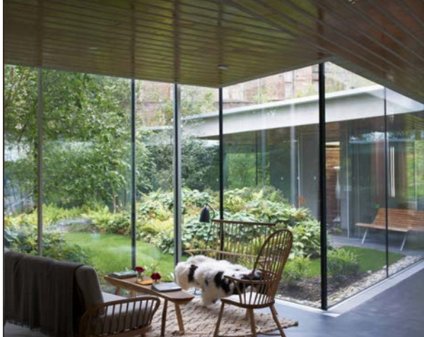
Figure 50: floor-to-ceiling curtainwall at Maggie's Gartnavel brings ample natural light (OMA; edit Braden Reid)
