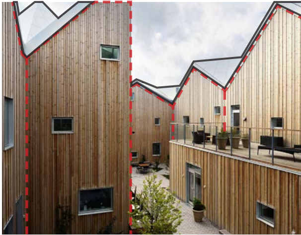
Figure 25: multiple smaller structures of the CCCH, tied together with a singular sculptural roof (NORD Architects; edit Braden Reid)
