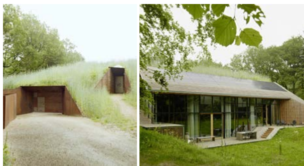
Figure 34: (L) Dutch Mountain House entrance view; (R) walkout plan on opposite elevation (ideasn.com)
