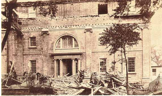
144. Destruction to MUSC after the Earthquake of 1886
