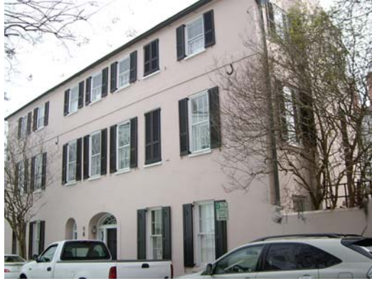
Figure 13: East Façade of 1 Tradd Street: note the operable shutters and storm windows. Photo by author.
