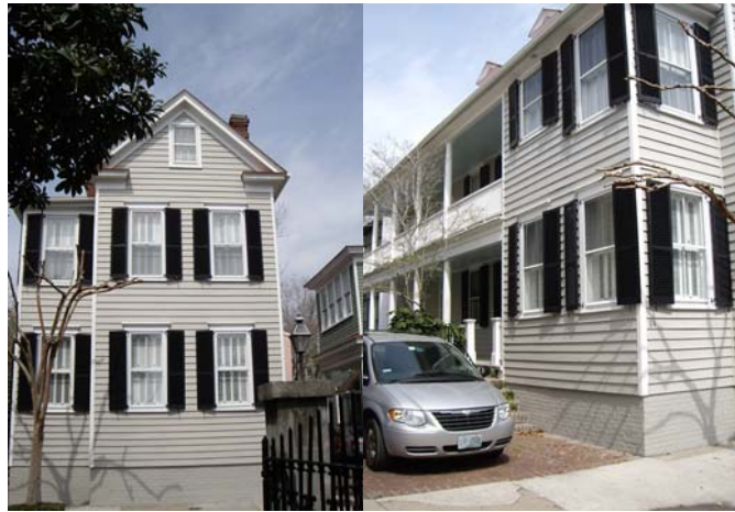
Figure 18: 84 Tradd Street has an enclosed crawl space, which is vented away from the street. Photo by author.
