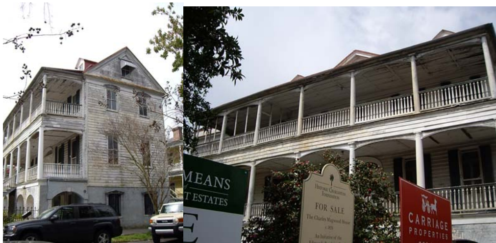
Figure 9: East and South Facades of 63 Smith Street. Photo by Author.
