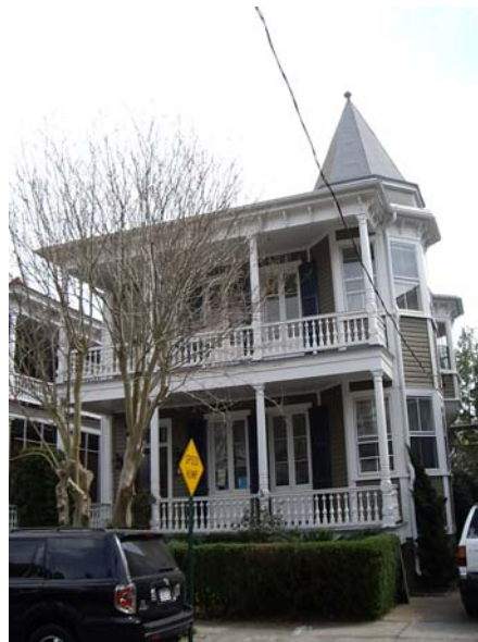
Figure 21: The French-door style windows combined with the shade of its porches once provided much-needed ventilation in its hot climate. Photo by author.
