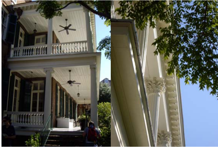
Figure 1: Porches, operable windows and shutters, and large cornices are all inherent energy saving features of historic structures. Photos by author.
