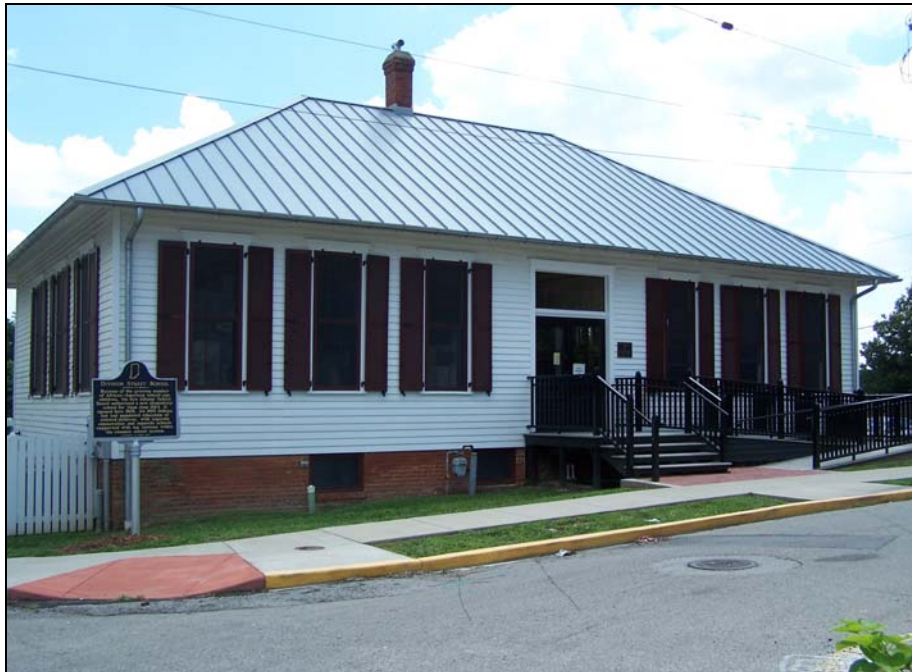
Figure 7: Division Street School after restoration, June 2006. Photograph by Sandi Feaster.
