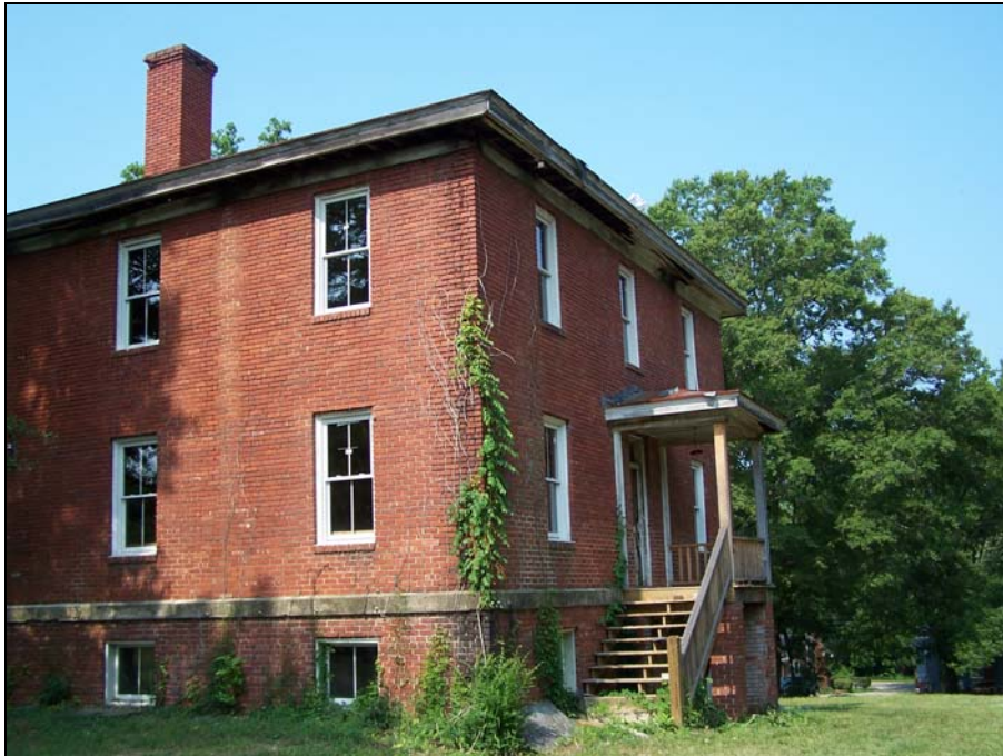
Figure 14: Rear of Kumler Hall, July 2006. Photograph by Sandi Feaster.
