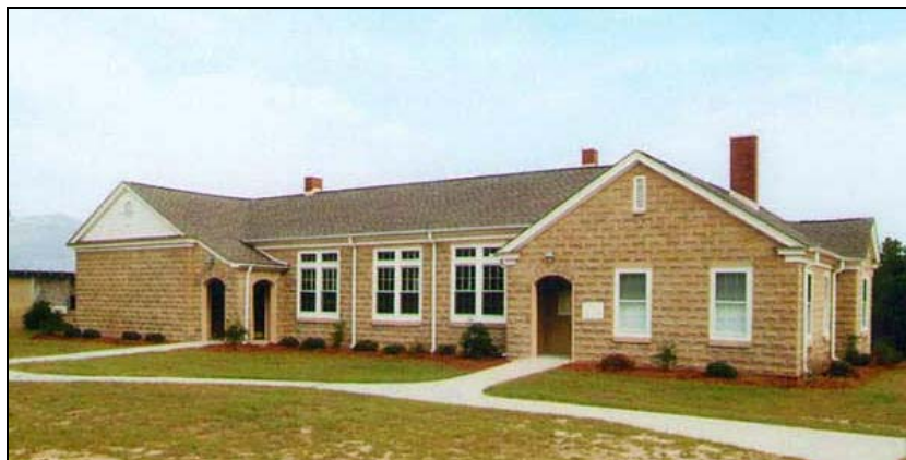
Figure 23: Biddle Hall after restoration. Photograph from South Carolina Department of Archives and History.
