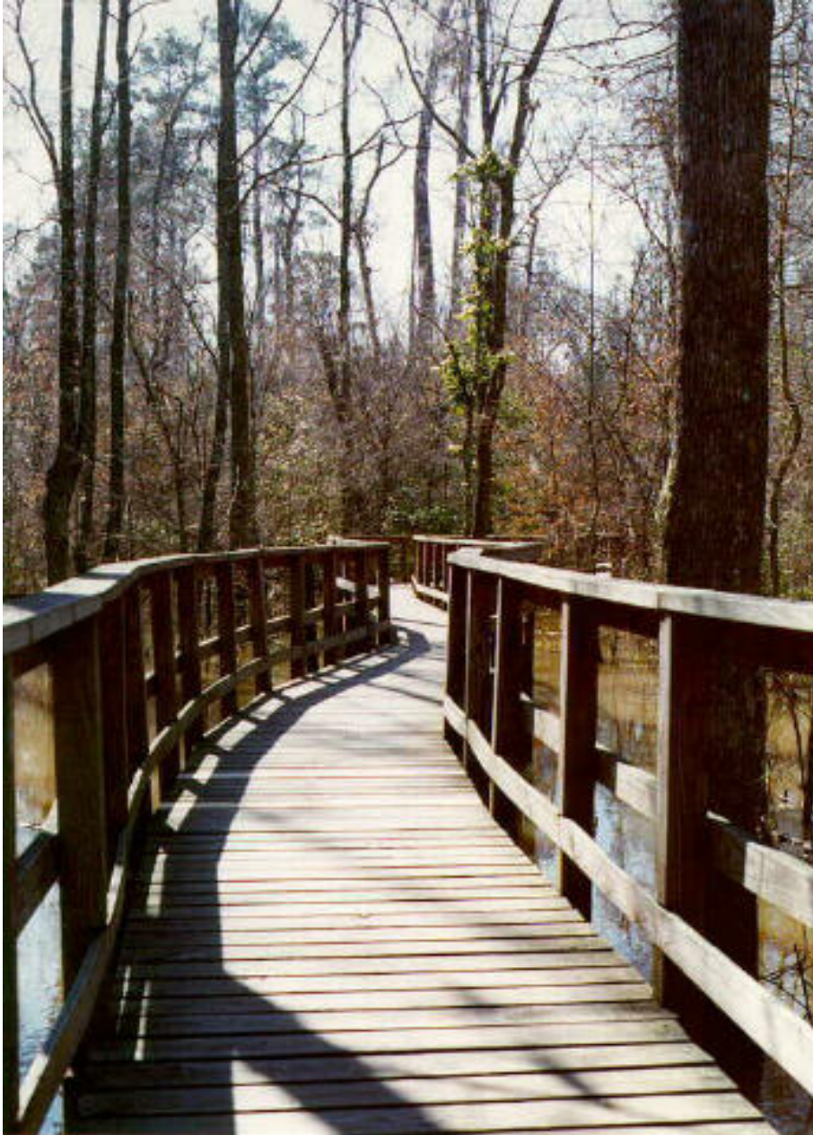
Figure 12. Example of a raised boardwalk traversing a wetland.
