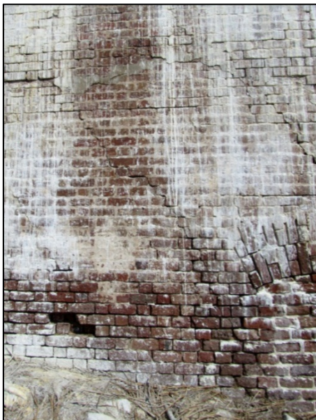
Figure 7.12 Showing diagonal fractures
