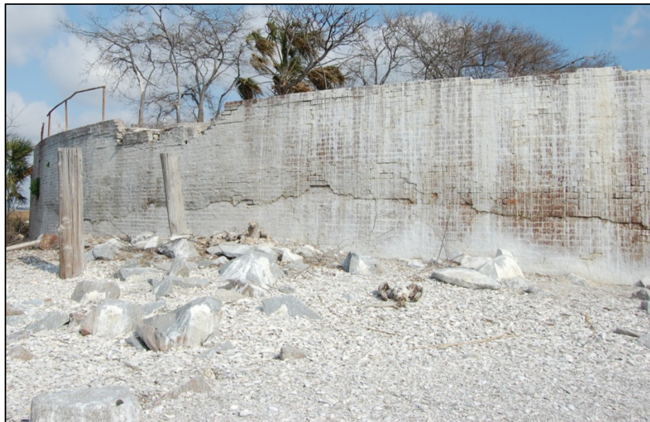
Figure 7.10 Showing major horizontal fracture
