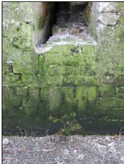
Figure 7.2 The highest proliferation of moss and microflora, at the base of the wall
