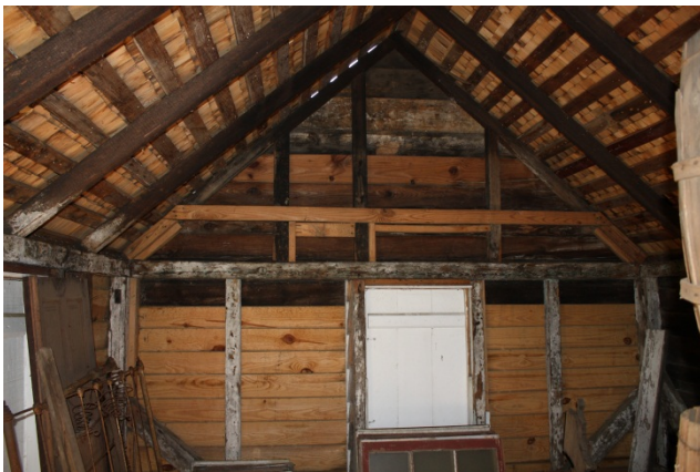
Figure 54: West wall, interior view, MSH-2.
