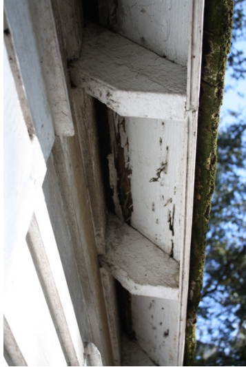
Figure 32: Underside of eaves, MSH-1
