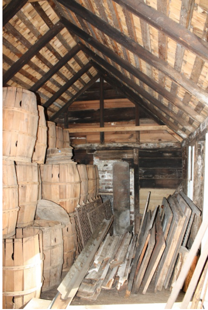
Figure 53: East wall, interior view, MSH-2.
