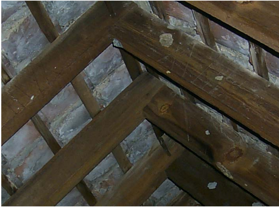
Figure 3.9. Rafters joined by mortise and tenon. Photo by author.
