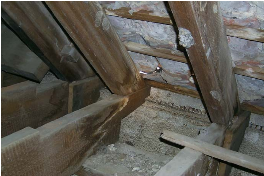
Figure 3.8. Mill sawn framing in attic of church. Photo by author.
