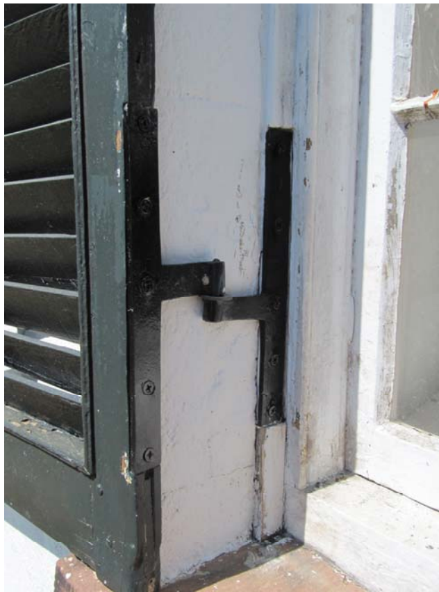
Figure 3.4. Cast hinges supporting louvered shutters. Photo by author.
