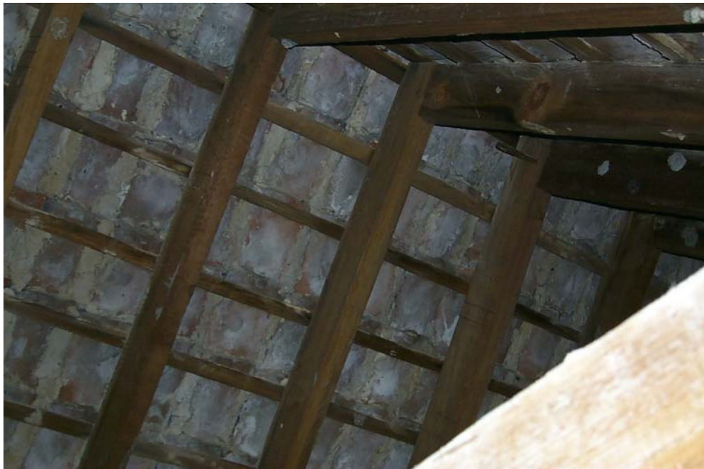
Figure 3.10. Photo of attic depicting sheathing supporting the pantiles. Photo by author.
