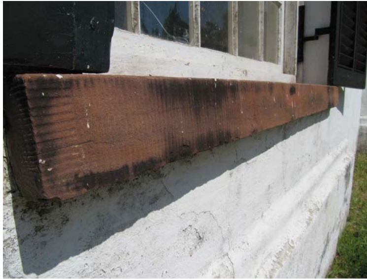
Figure 3.5. Tooled sandstone sills. Photo by author.
