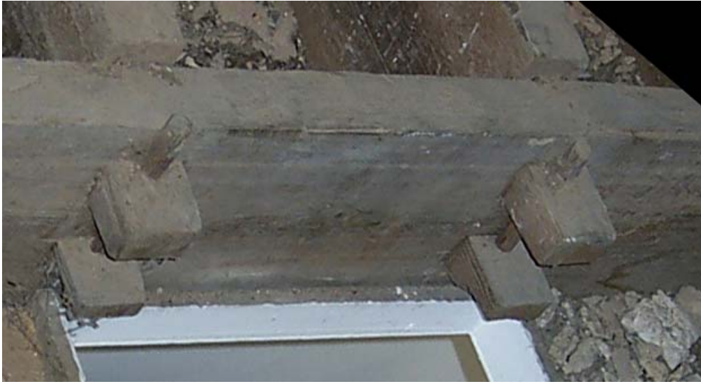
Figure 3.11. Double tenoned outlookers in attic of church. Photo by author.
