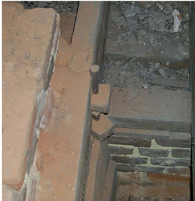
Figure 3.12. Dragon beams in corners of attic. Photo by author.
