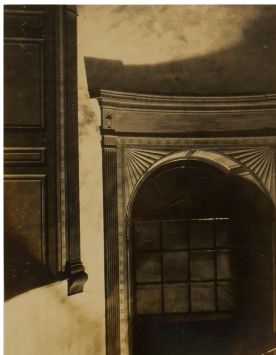
Figure A.12: Window surround. Photographer Albert Simons.
