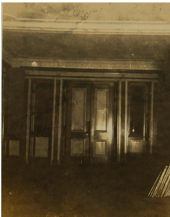
Figure A.11: Interior door. Photographer Albert Simons.
