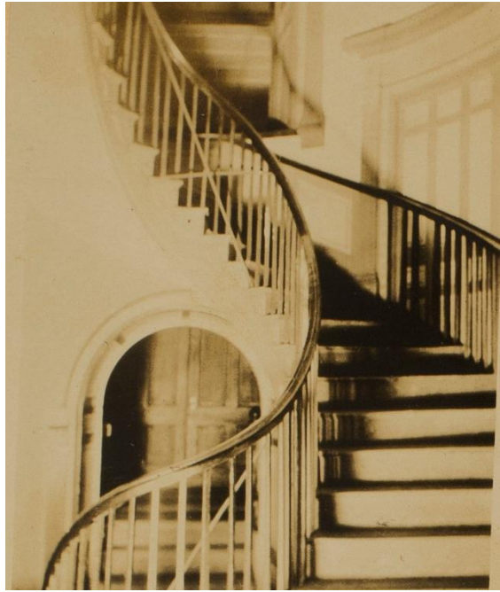
Figure A.15: Stairwell. Photographer Albert Simons.
