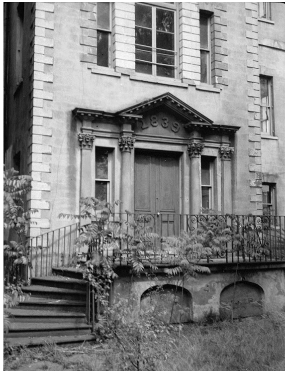
Figure 2.15: The entablature of the entrance. From loc.gov , Thomas Ratcliffe House, 24 George Street, Charleston, SC
