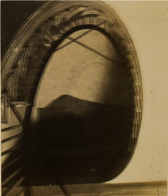
Figure A.14: Stairwell. Photographer Albert Simons.
