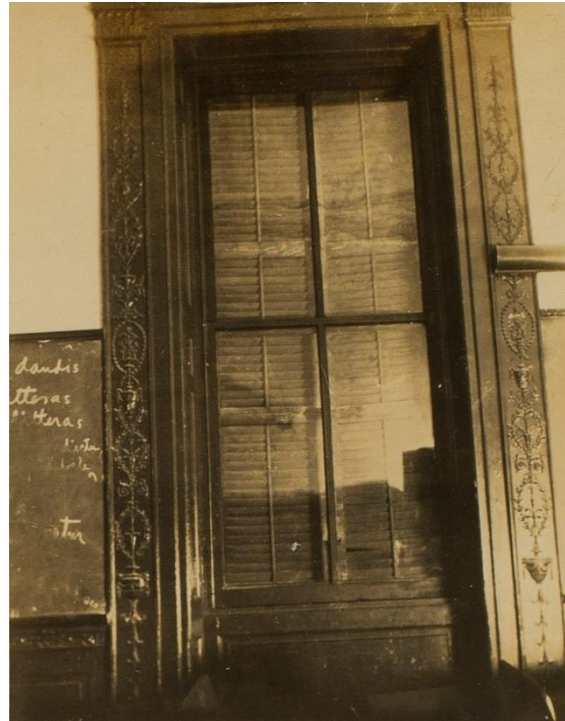
Figure A.21: Window details. Photographer Albert Simons.
