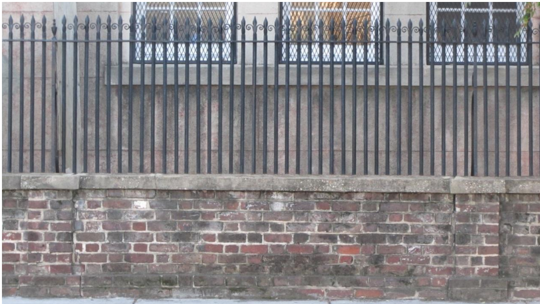
Figure B.1: One section of the historic wrought ironwork.
