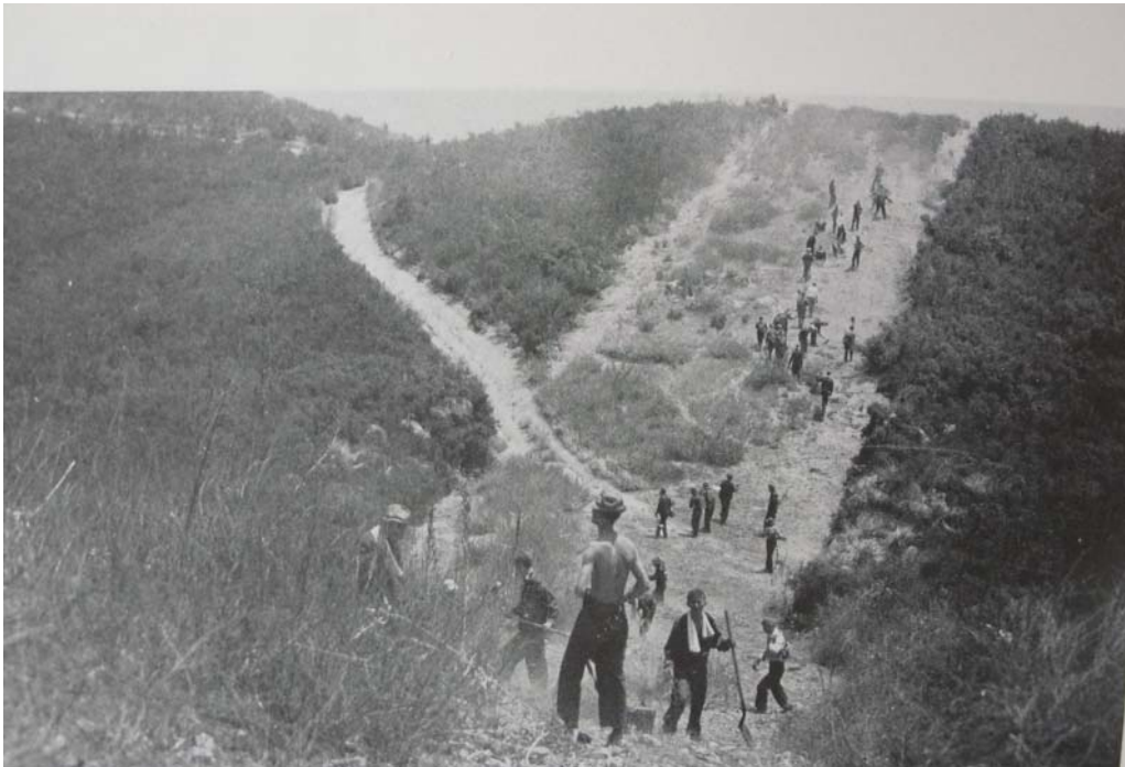
Figure 4.4: CCC men building a fire break to aide in fire suppression. From Stan Cohen, The Tree Army: A pictorial history of the Civilian Conservation Corps, 1933-1942 .
