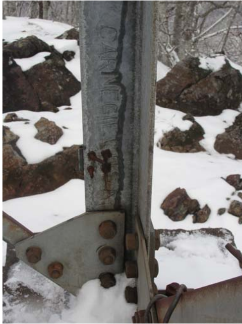
Figure 6.5: Carnegie stamp on steel tower at Shuckstack. Photo by author.
