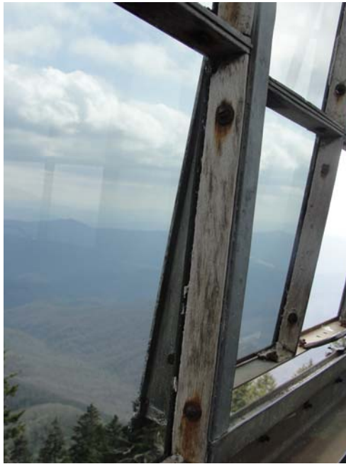
Figure 6.7: Steel cab atop Mount Sterling tower. Photo by author.
