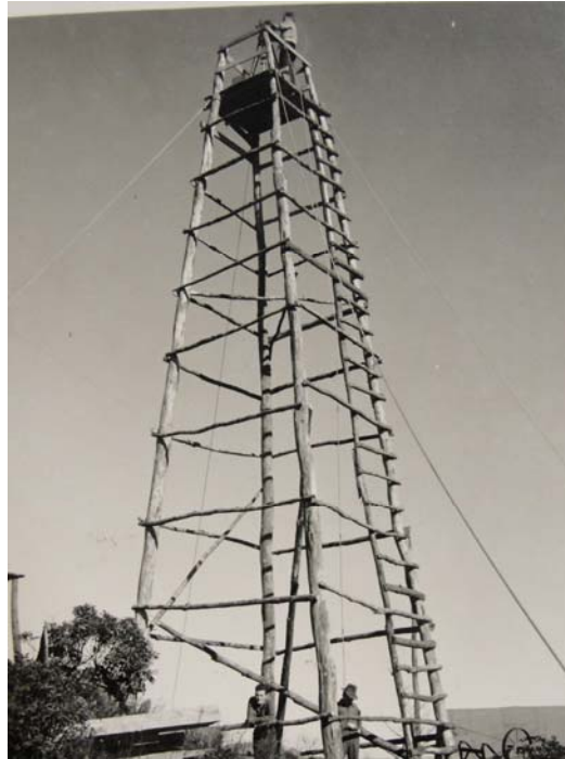
Figure 6.3: Temporary tower constructed at proposed tower site in order to obtain panoramic photographs. Photo by L. M. Moe, November 1935. Courtesy of GRSM Library.
