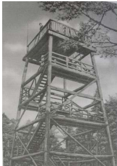
Figure 6.22: Timber tower at Clingman's Dome, 1937. Courtesy of GRSM Library.
