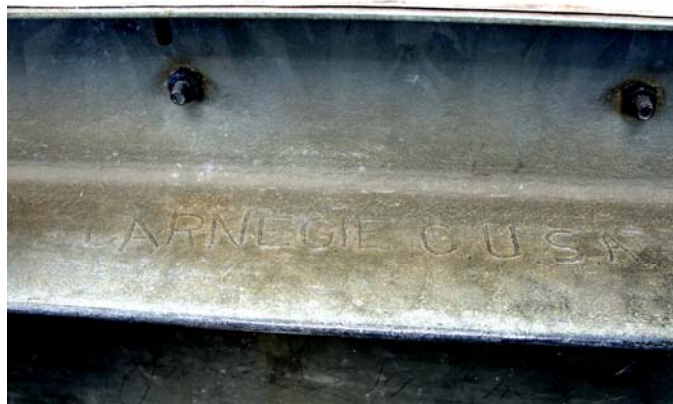
Figure 6.8: Carnegie stamp on steel member of Mount Sterling tower. Photo by author.
