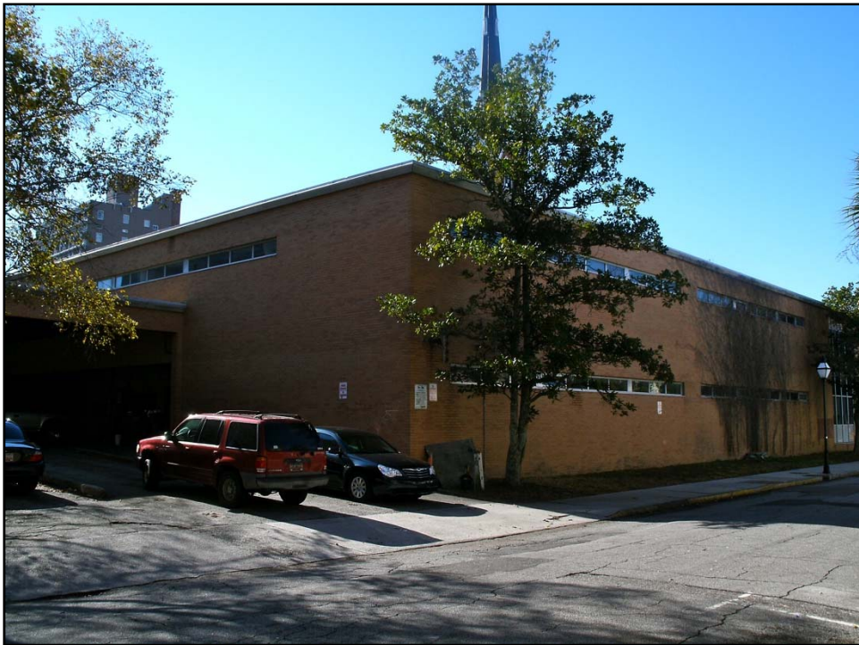
View from Hutson Street
