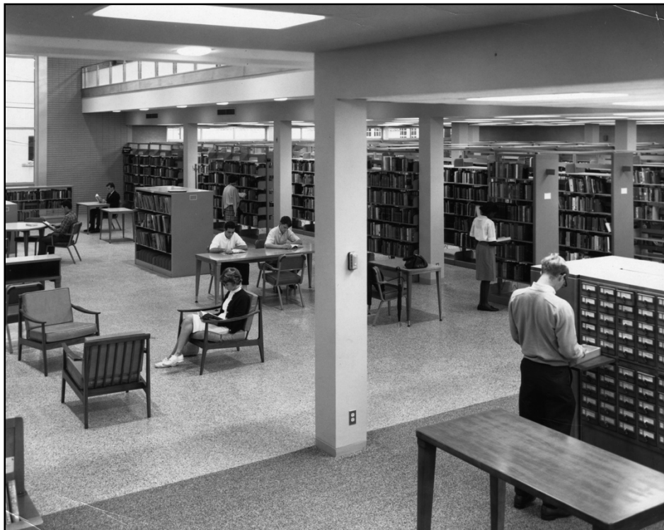
View of Charleston County Library interior
