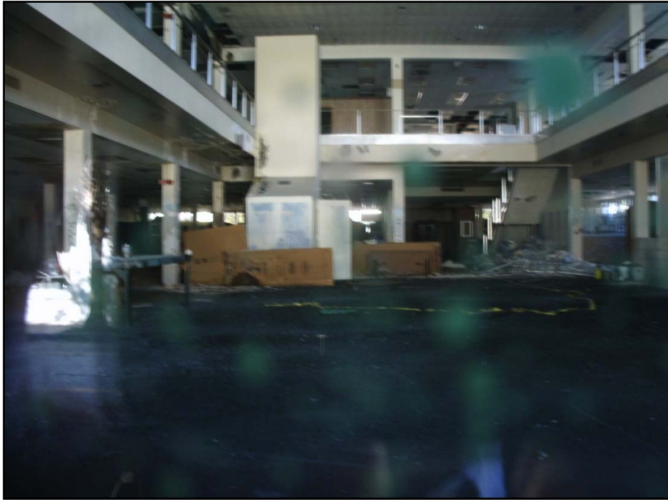
Interior view from Hutson Street
