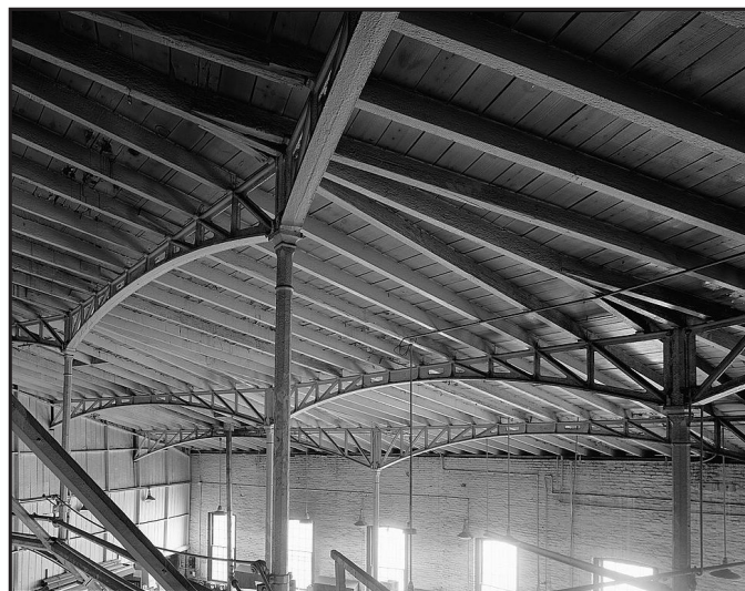
Figure 4.2: West Virginia Railroad Station showing cast iron columns and trusses. (courtesy of the Library of Congress)
