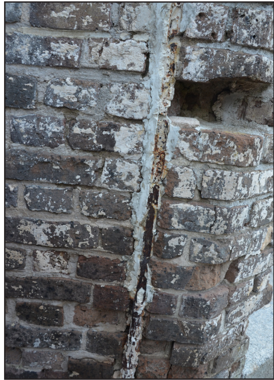
Figure 8.7 Gas piping fragments found along the Gorge Wall. (photo by author)
