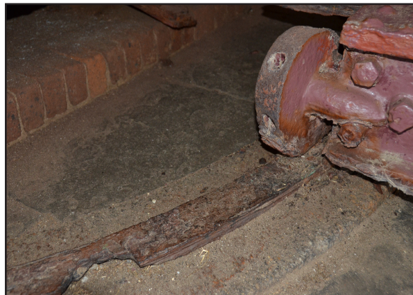
Figure 8.1: Traverse rails in Right Face with no visible paint layers. (photo by author)
