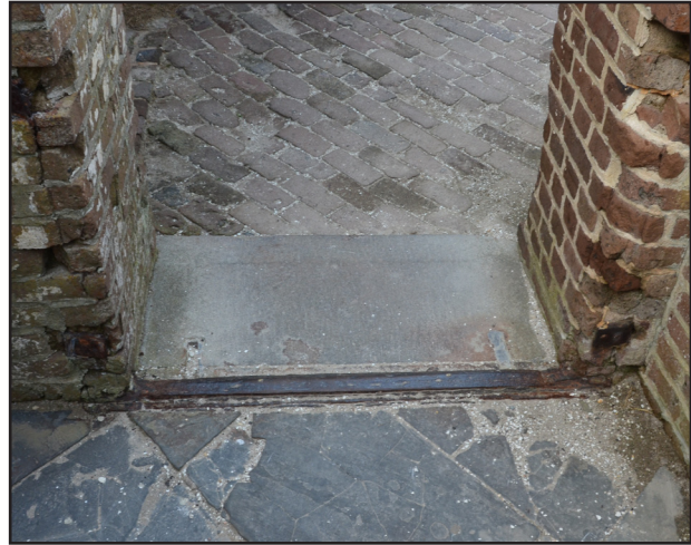
Figure 4.30 (left) Door hardware remanents from original magazine along Gorge Wall
