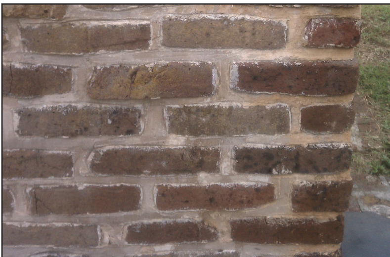
Figure 6.7 Locally-made Charleston grey brick that is common through the fort. (photo by author)
