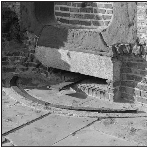
Figure 4.21: HABS image showing intact pintle along Left Face. While the exact casemate is unknown, this pintle is no longer in existence. (courtesy of the Library of Congress).
