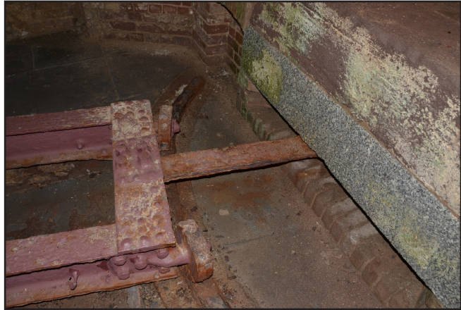
Figure 6.12 Granite Lintel over pintle tongue in Right Face. (photo by Author)
