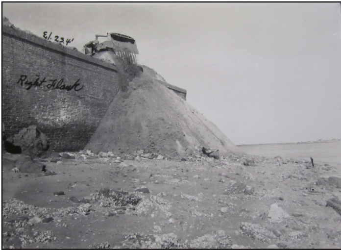
Figure 4.12 Excavator dumping excavated dirt over the scarp wall during the 1950s excavation (courtesy of Fort Sumter National Monument).
