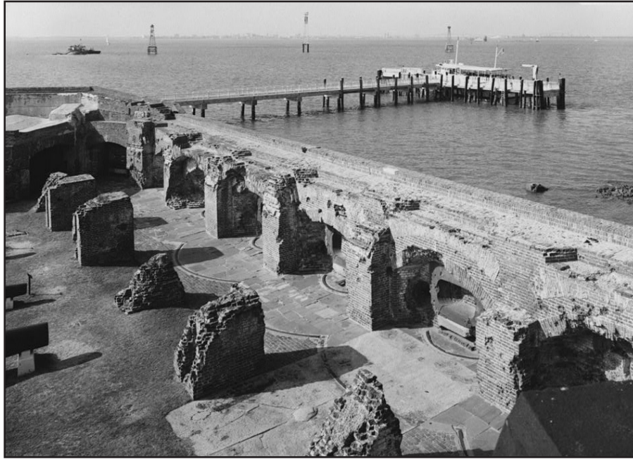
Figure 4.15 Left Face showing existing traverse rails from Historic American Building Survey Documentation. (courtesy of the Library of Congress)
