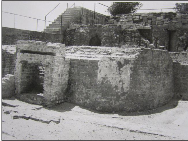
Figure 4.29 1956 Excavation Report image detailing fireplace as found. (courtesy of Fort Sumter National Monument)
