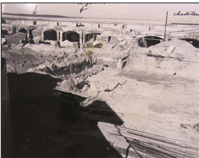
Figure 4.14 Left Flank and parade ground being excavated during 1956 excavation (courtesy of Fort Sumter National Monument)
