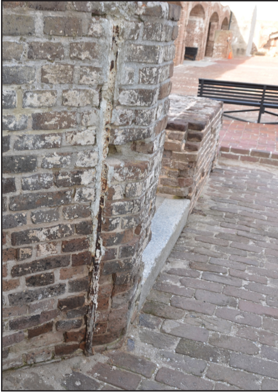
Figure 4.32 Little Gas Piping remains from the Confederate Installation. Photo by author.
