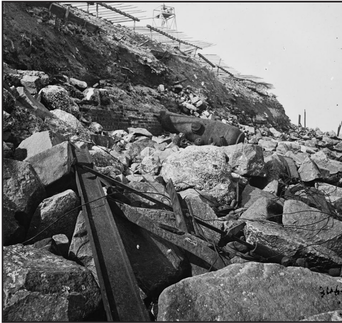
Figure 4.10: After the destruction of the barracks, the I-beams served a second life as support for a barbed wire fence to ward off a potential land invasion. (courtesy of the Library of Congress)
