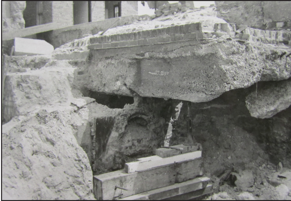
Figure 7.1 Fireplace basket underneath concrete foundations during the 1950s excavations. (courtesy of Fort Sumter National Monument)
