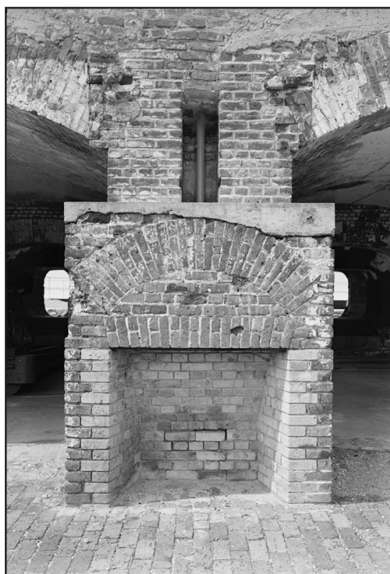
Figure 4.23 HABS image of Left Flank Fireplace. (courtesy of Library of Congress)
