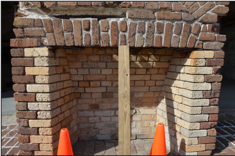
Figure 6.5: Yellow firebrick at Fort Sumter. Likely, this firebrick was brought to the fort at a later date after the Civil War. (photo by author)
