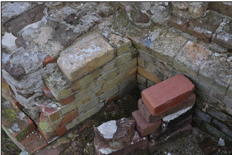
Figure 6.6 Finer quality extruded brick found in the area around the Officer's Quarters. (photo by author)
