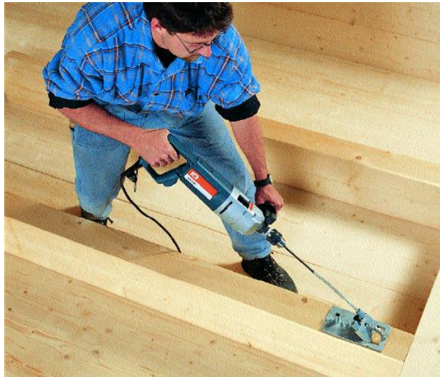
Figure 2.10: Self-Tapping Screw Used as End of Beam Connection (SFS Intec, Inc.)
