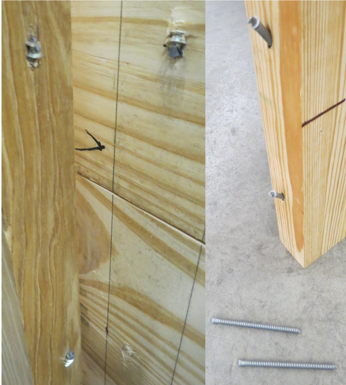
Figure 4.49: Typical Screw Failure Modes (ASSY on Right and SFS Intec on Left)
