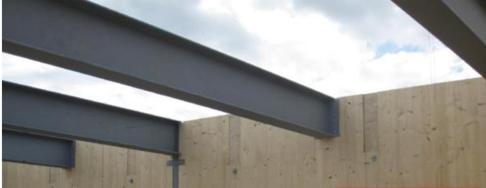
Figure 2.12: Steel Beam-to-Wood Connection (Wallwork)
