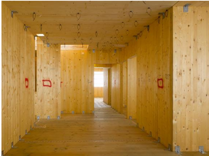
Figure 2.5: Structure of CLT Building (Waugh Thistleton)
