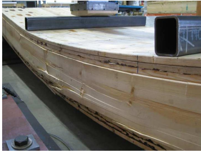
Figure 2.16: Web Bending Stress Failure Caused by Lack of Composite Action (Chen)
