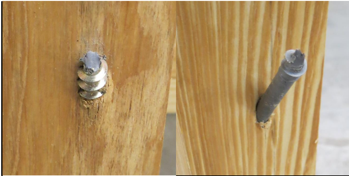
Figure 4.50: Typical Rupture of Screw (ASSY on Right and SFS Intec on Left)
