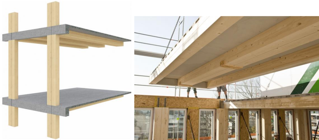
Figure 2.14: Life Cycle Tower Floor Panels (Rhomberg Group)
