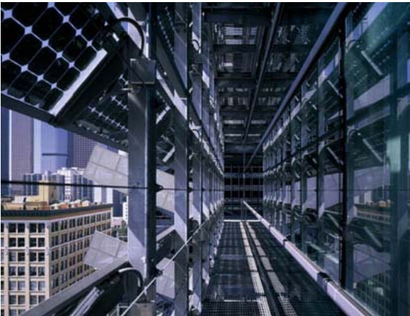
Fig. 36 CalTrans Building by Morphosis, Double Wall System
