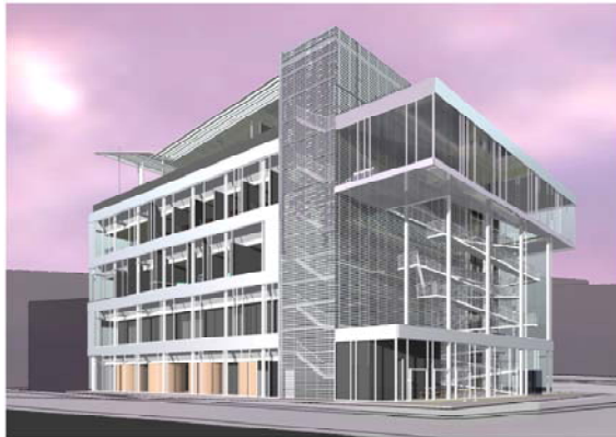
Fig. 76 Overall Building Form, Showing Wrapping of Interstitial Spaces
