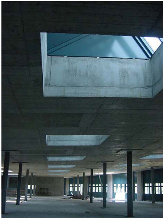
Fig. 31 INO Hospital, light wells
