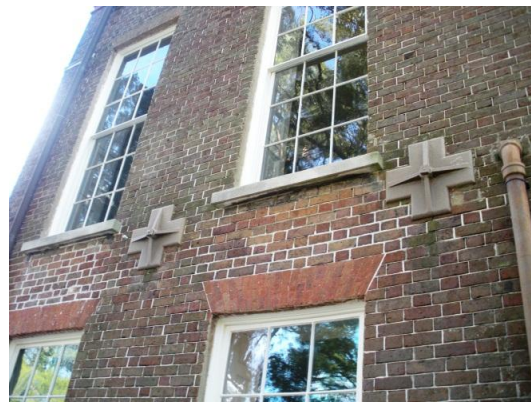
Figure 4.22: The Nathaniel Russell house features three different tie rod anchor plate forms: Top Left: Plain, circular anchor plate on the front façade. Bottom Left: Circular anchor plate with molded profile on the front façade. Right: Cruciform shaped anchor plates on the north façade. (Photos taken by author)
