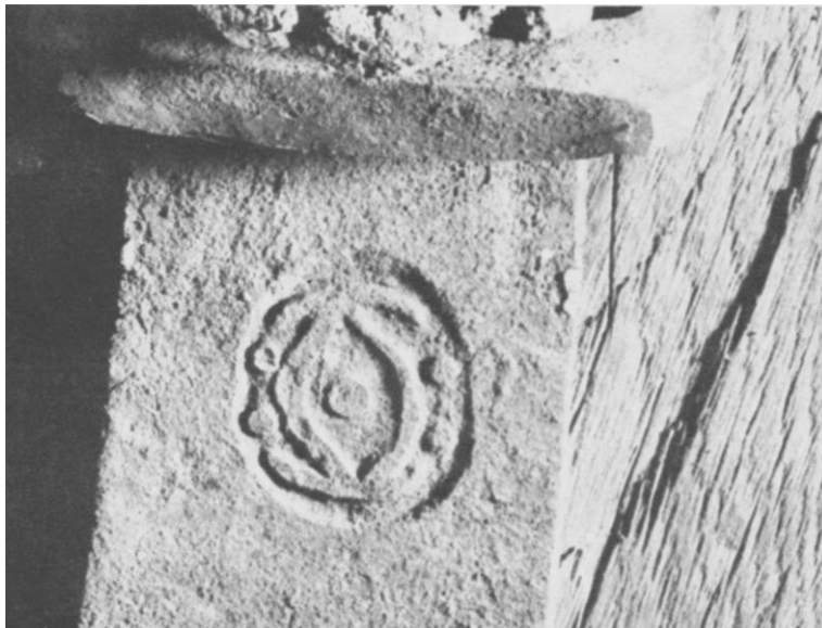
Figure 4.12: "Horseshoe" iron mark at Christ Church, Lancaster County, Virginia (1732) (Source Carlton, "Marks on the Iron Stirrups, APT , Vol. VII No. 1)
