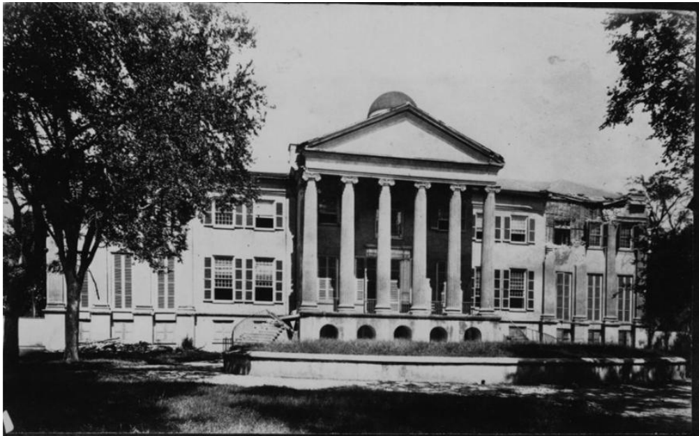
Figure 4.31: South façade of Randolph Hall after the Charleston Earthquake of 1886. Damage to east wing is visible on right. Both wings were eventually removed and reconstructed. (Source: Low Country Digital Library; < http://lowcountrydigital.library.cofc.edu >)
