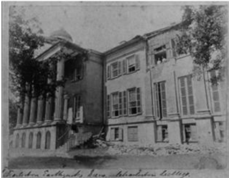
Figure 4.32: Earthquake damaged south façade of Randolph Hall. Damage to east wing is visible on right and evidence of the portico pulling away can be seen on the left. (Source: Low Country Digital Library; < http://lowcountrydigital.library.cofc.edu >)
