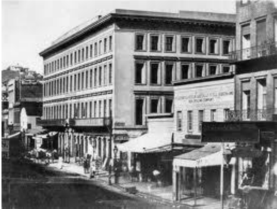
Figure 2.12: The Montgomery Block in San Francisco, CA, erected with iron reinforcement probably designed to resist earthquakes and settlement. (Source: Tobriner, Bracing for Disaster , 17)
