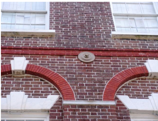
Figure 4.22: The Nathaniel Russell house features three different tie rod anchor plate forms: Top Left: Plain, circular anchor plate on the front façade. Bottom Left: Circular anchor plate with molded profile on the front façade. Right: Cruciform shaped anchor plates on the north façade. (Photos taken by author)
