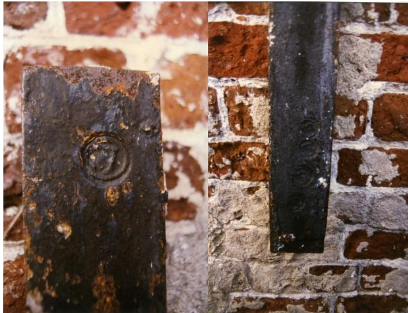
Figure 4.7: Maker's marks stamped onto the iron anchor plate arms. Images were taken during the 1996 restoration. (Photo courtesy of Richard Marks Restoration, Inc.)
