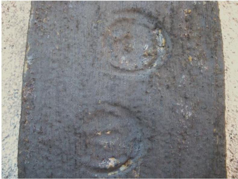
Figure 5.2: Evidence of maker's marks & paint deterioration on the northeast anchor plate arm. (Photo taken by author)
