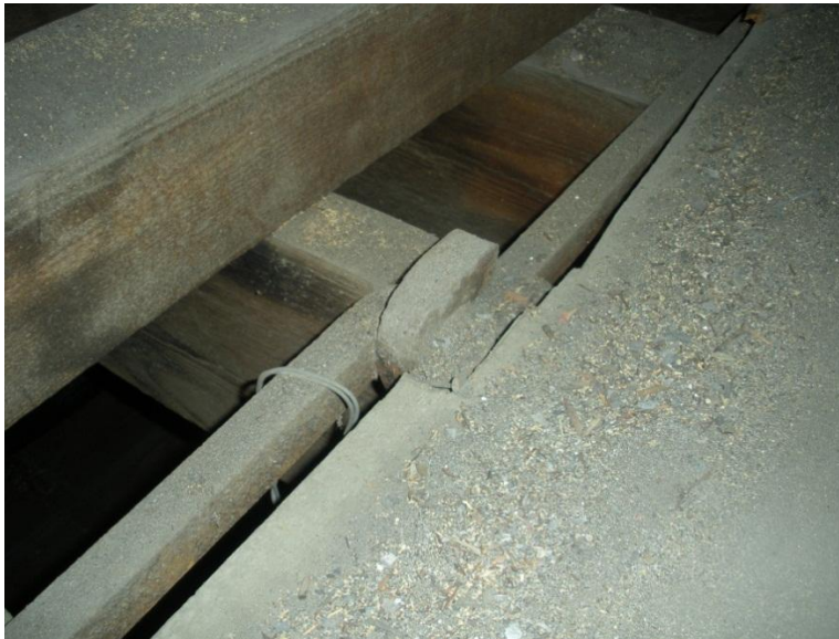
Figure 4.30: Center hook connection. (Source: Photo taken by author)
