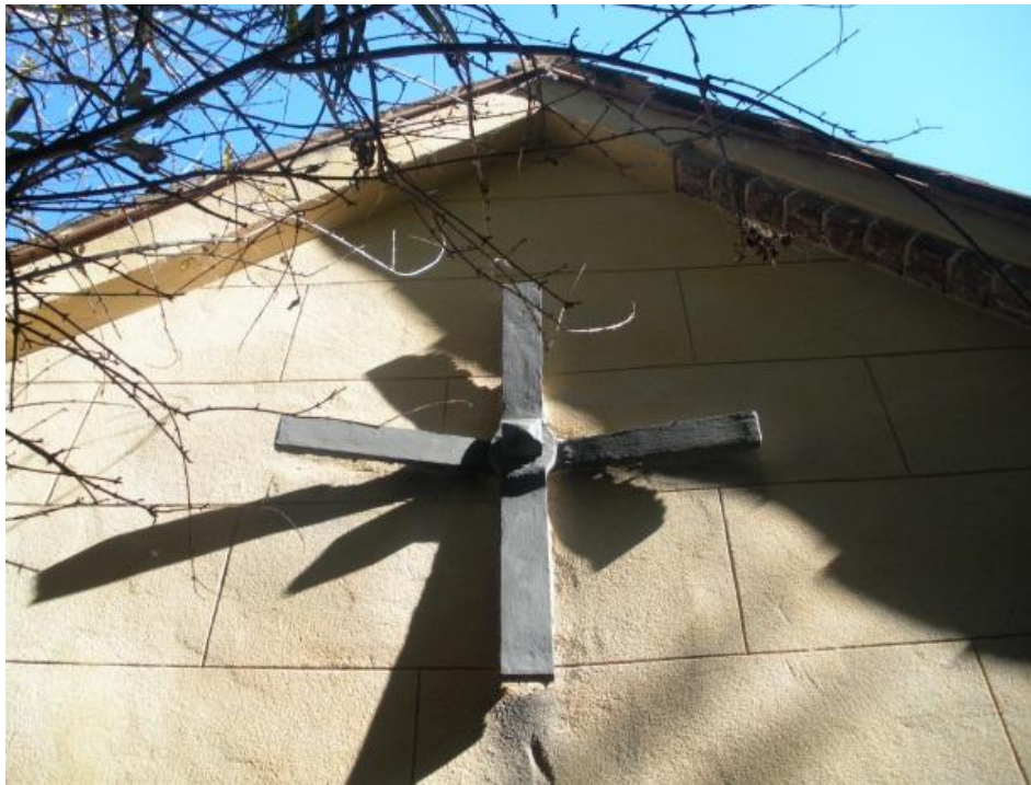
Figure 4.4: Exterior anchor plate on north-west gable. (Photo taken by author)
