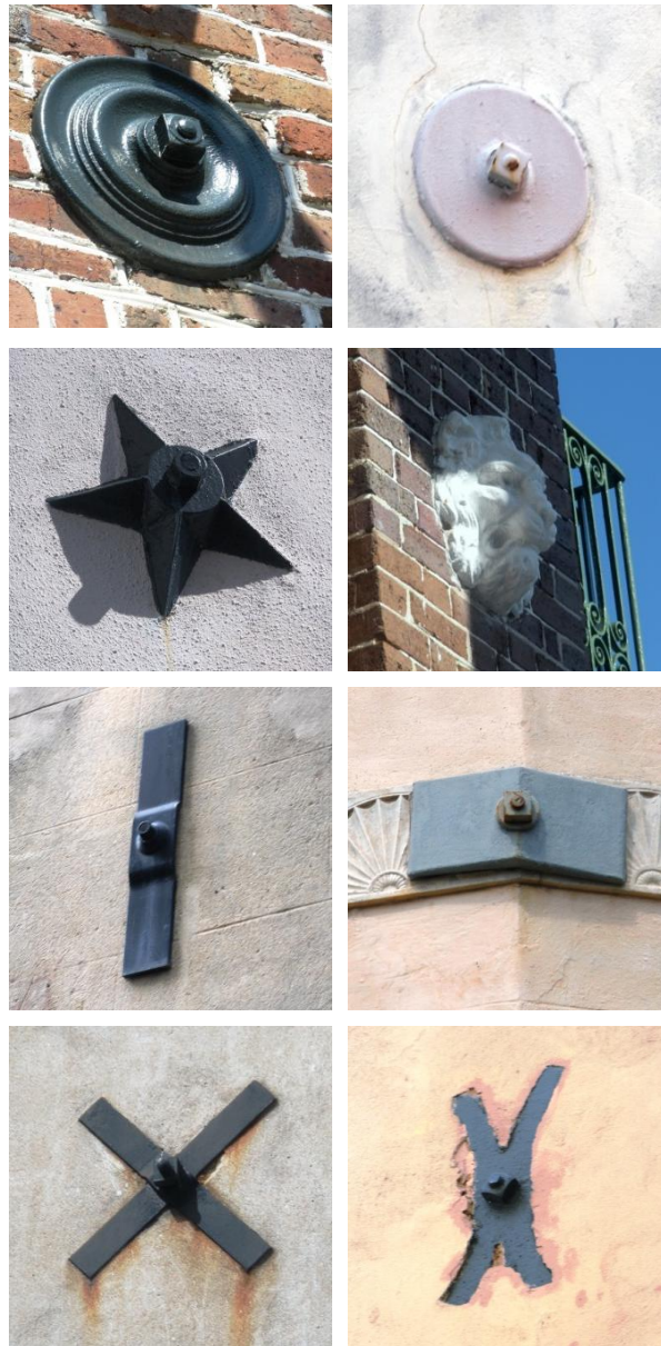
Figure 3.8: Various forms of ‘earthquake bolt’ patrix plates observed around the city of Charleston (All photos taken by author).
