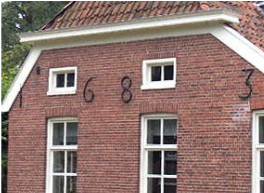
Figure 2.6: Dutch short wall anchors with decorative exterior attachments revealing the date of construction in Great Yarmouth, Norfolk. (Source: Reynolds, Transmission and Recall , PhD diss.)
