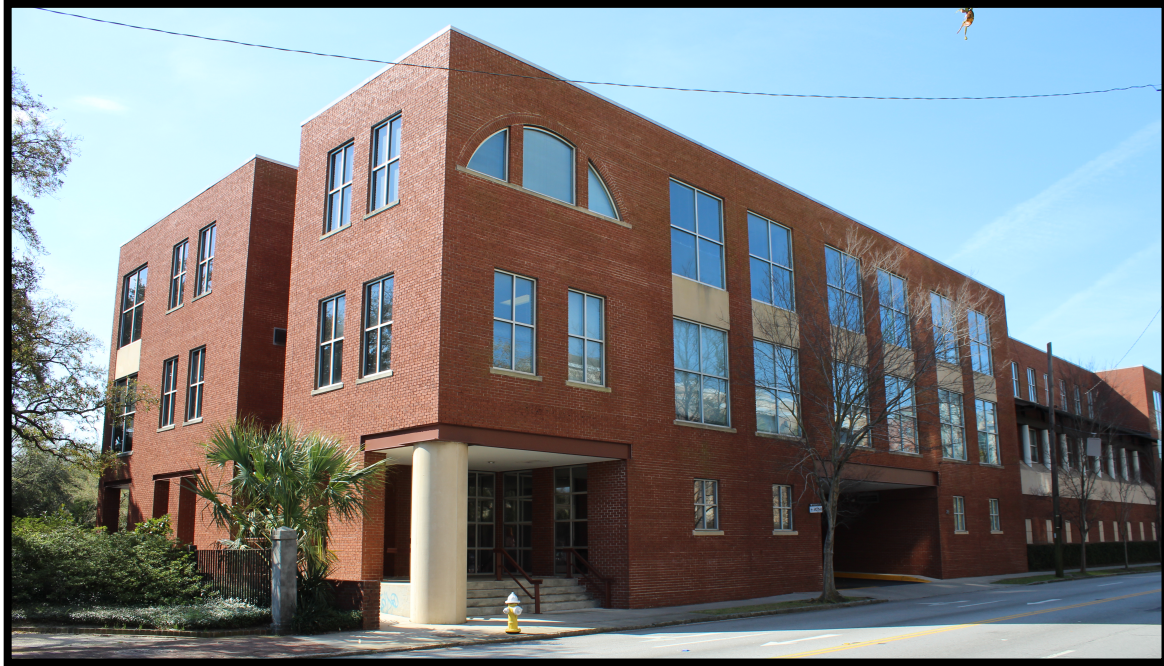
Figure 5.6: Cannon Park Place, Northwestern Facades, 261 Calhoun Street; author's image.
