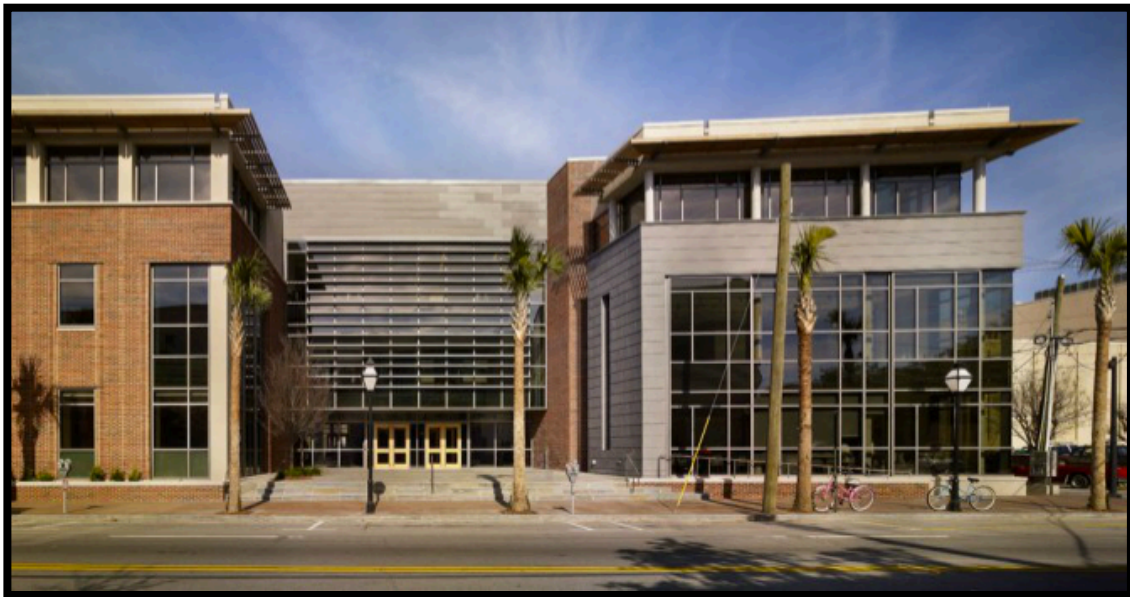
Figure 4.8: College of Charleston Science Building; image courtesy Ballinger Architecture, http://www.ballinger-ae.com/#/projects/228 .
