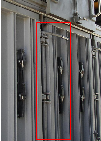
Figure 4.5: Current Baling System Locking Mechanism
