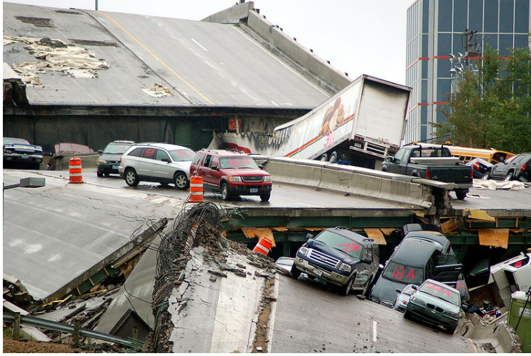
Figure 1.4: The I-35W Mississippi River bridge collapse. Picture taken by Kevin Rofidal, United States Coast Guard.
