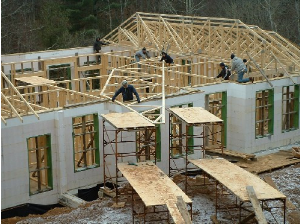
Figure 2.1 Offsite Preassembled Roof Trusses (Courtesy of Timer Engineering, UK)
