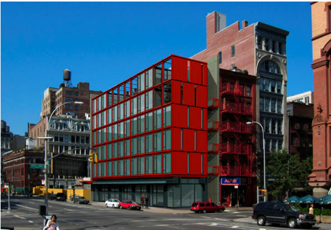
Figure 2.4 Modular building at Lafayette Street, New York City, United States (Courtesy of Urban Space Management, Inc.)
