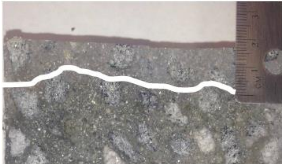
Figure B.2. Chloride penetration after two month
