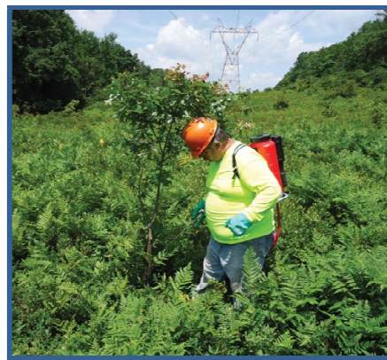
Herbicide application within utility right-of-way using backpack sprayer.
