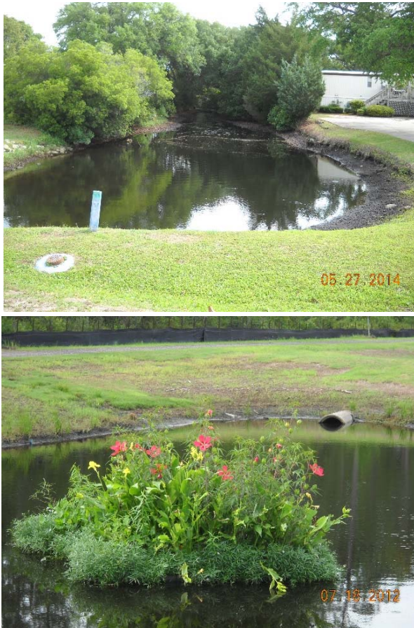
Figure 2. Floating treatment wetlands and target site at in-line detention pond.
