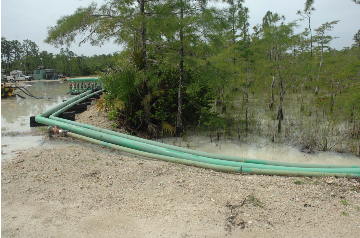
Figure 3.1: Image at the exit road for pad #5 at Collier Resources Company's Raccoon Point oil field. The image was take after a large rainfall event and shows significant water accumulation on the surface of the pad and a small breach in the levee (near the front flowline) that is draining turbid water into the adjacent cypress swamp. This image also shows flowlines coming into contact with surface water in the wetland (Photo by Jerome Jackson).
