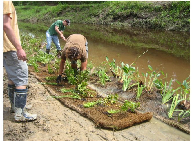
Figure 5. Installation of pre-rooted aquatic carpets.
