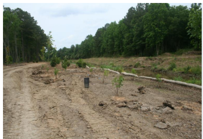
Figure 2. (a) Left hand photograph shows steepened banks of Crabtree Canal prior to restoration. (b) Right-hand photograph shows restored floodplain during planting. Erosion control logs are located at top of bank in the aquatic zone.
