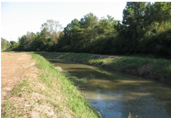
Figure 2. (a) Left hand photograph shows steepened banks of Crabtree Canal prior to restoration. (b) Right-hand photograph shows restored floodplain during planting. Erosion control logs are located at top of bank in the aquatic zone.
