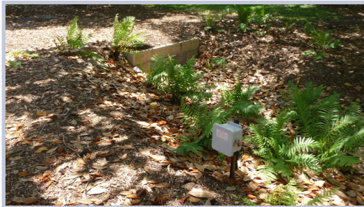
A parkway in Aiken reconstructed with a bioswale and wireless monitoring equipment.
