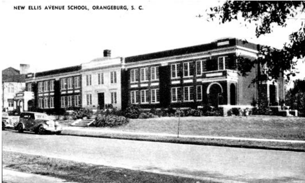
The “new” Ellis Avenue School, built in the early 1930s; I attended the first through third grades here.
