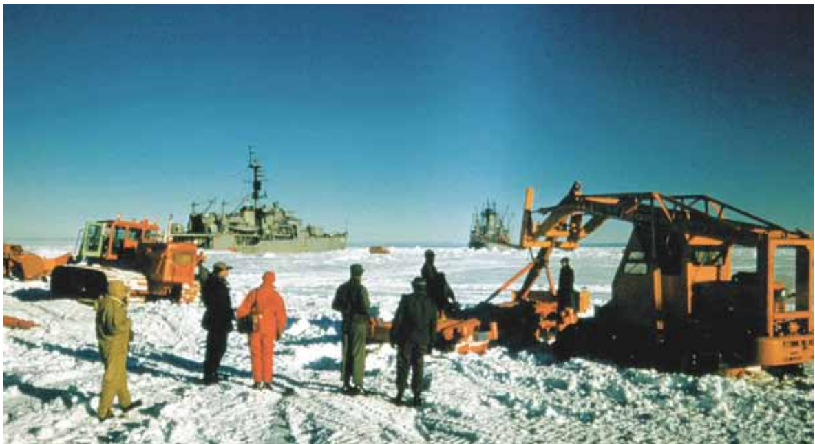
Fig. 1.1-8 U.S. Navy and construction personnel unload cargo on the Antarctic shore-fast ice during the U.S. "Deep-Freeze I" mission, 1955–1956, in preparation for IGY 1957–1957. (Photo: Rocky Milano)
