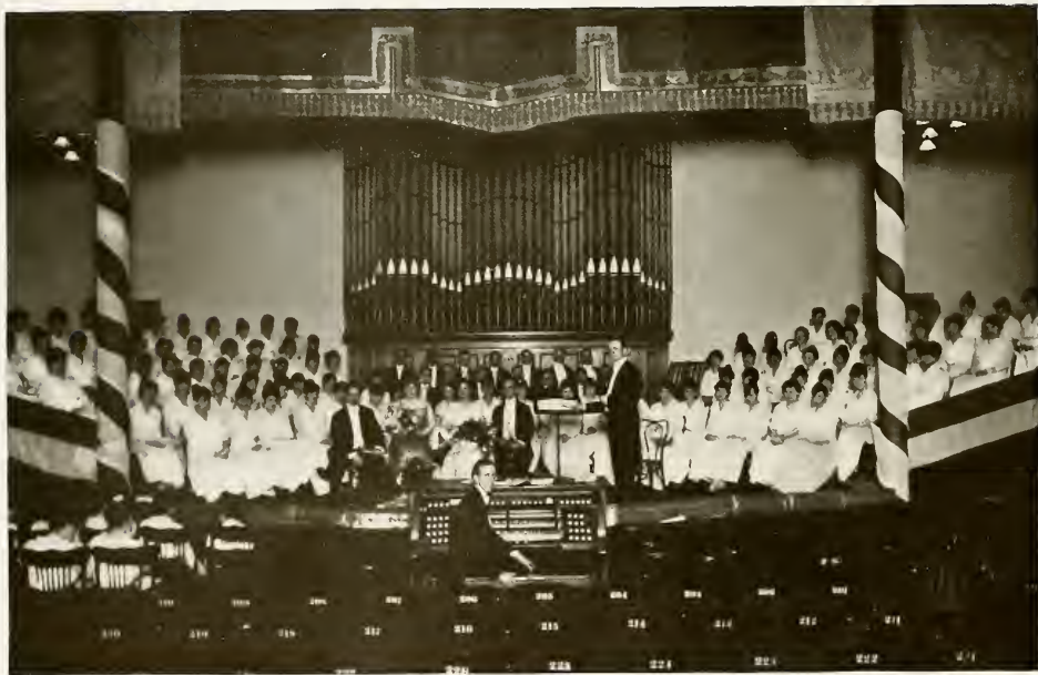
WARD-BELMONT CHORAL SOCIETY, ASSISTED BY SOLOISTS AND THE VANDERBILT UNIVERSITY GLEE CLUB IN A CONCERT PRODUCTION OF THE OPERA "MARTHA," UNDER THE DIRECTION OF MR. BROWNE MARTIN, WARD-BELMONT AUDITORIUM, APRIL 16.
