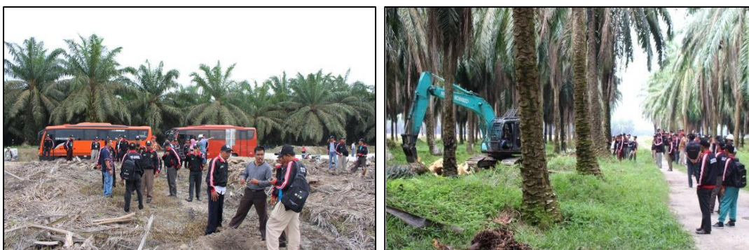
Figure 3 Training participants see the activities of land preparation for palm oil plantation replanting
