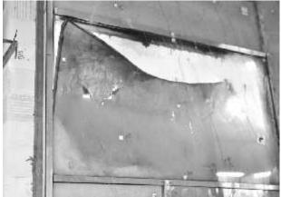
Fig. 8 IGU glass of EI90 type failure
