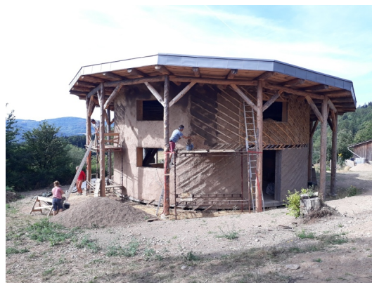
FIGURE 2. Building of family house from straw and earth in Klášterecká Jeseň.
