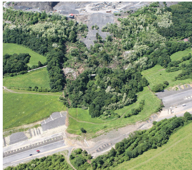
FIGURE 1. Picture of the landslide after collapse (summer 2013).
