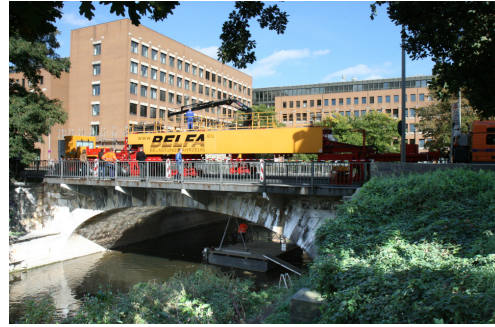
FIGURE 4. BELFA Test Loading of Stone Masonry Arch Bridge, Hanover
