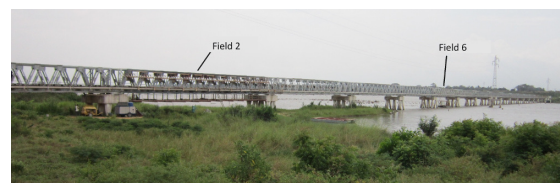
FIGURE 7. Steel Truss Bridge crossing the Lac Togo and tested fields
