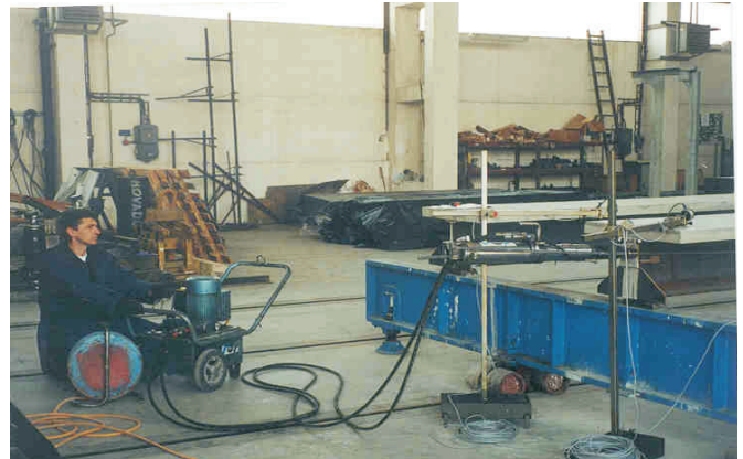
Fig. 3: Stressing of tendons by means of a hydraulic jack unit
