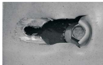
Fig. 9: Collapse mode of the connection from set C, temperature 200 °C
