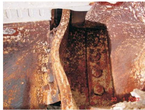
Fig. 11: a) Temperature distribution within the protected column during heating (after 30 min.) during cooling (after 120 min.) by Tempcalc code; b) local buckling of column flange E2
