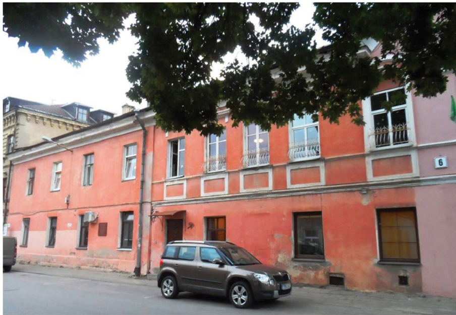
The building at 6 Plock Street where the Cancer Research & Clinical Centre was located (present state)
