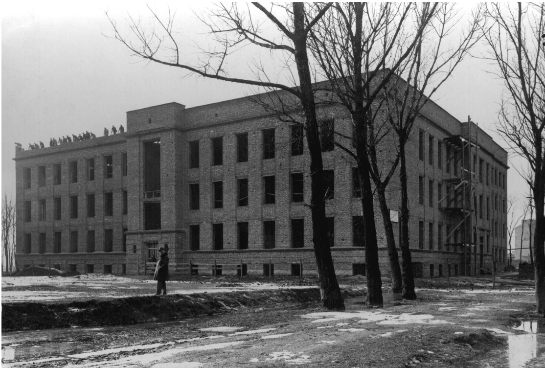
The Radium Institute under construction – main clinical building (March 15th 1927)
