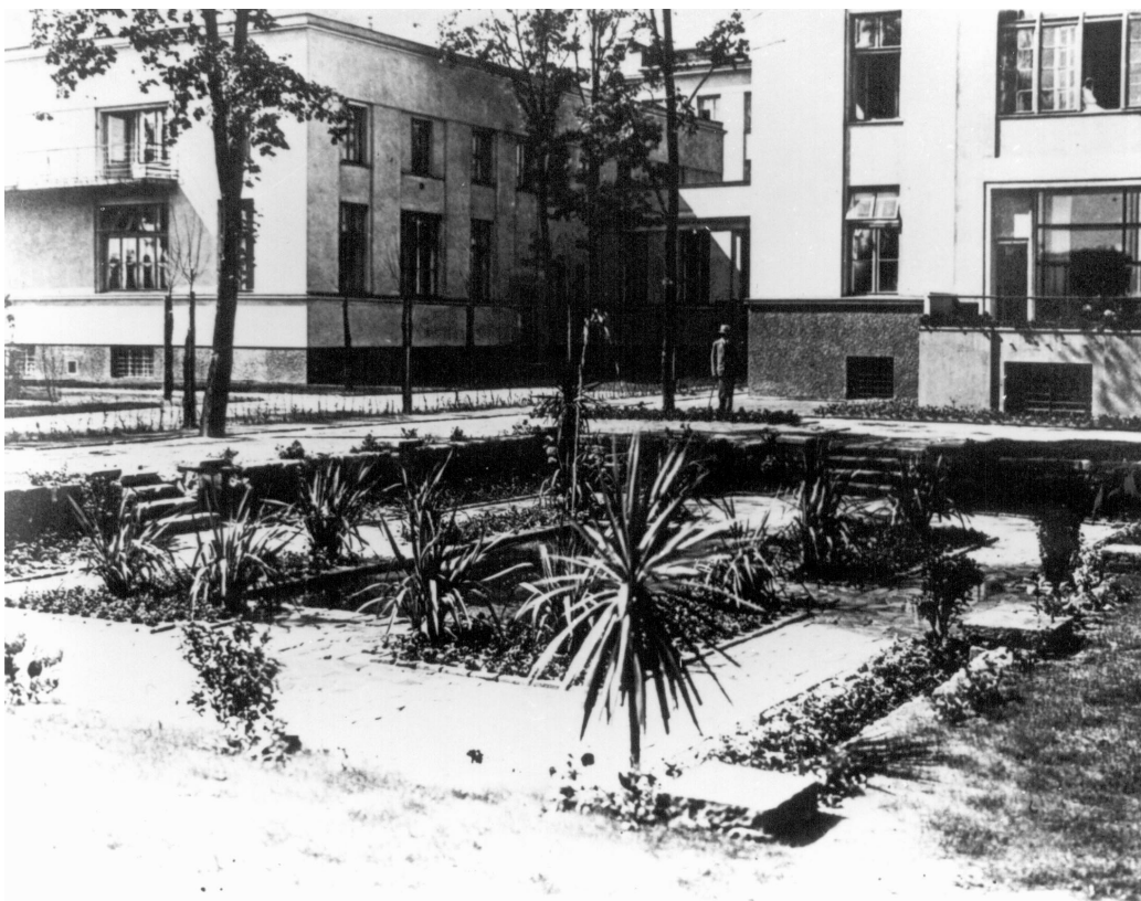
The clinical building seen from the research laboratories. The large window on the ground floor far right belonged to the apartment of Bronisława Dłuska, Maria's sister, who supervised the construction, and later the activities of the Institute. Maria stayed here when she came to open the Institute in May 1932
