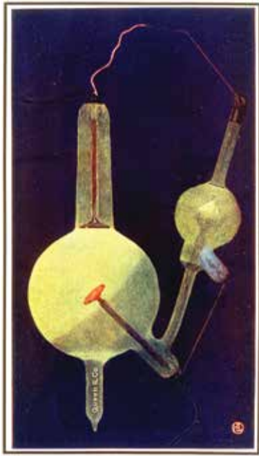
Figure 5. Self-regulating X-ray tube operating properly [1, 2]
