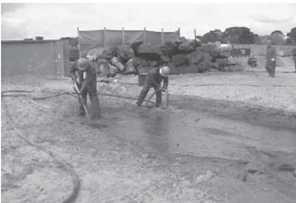
Figure 4. Removing buried pollutant
