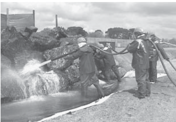
Figure 3. Cleaning riprap
