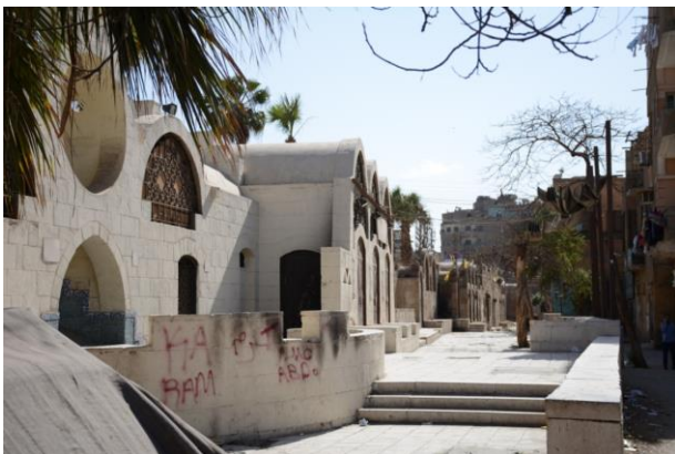
Figure 10: View from Abu-ElDahab Street Entrance, Authors, 2018.
